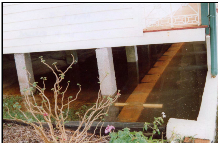
Figure 20 Water below lake frontage residence June 2005
