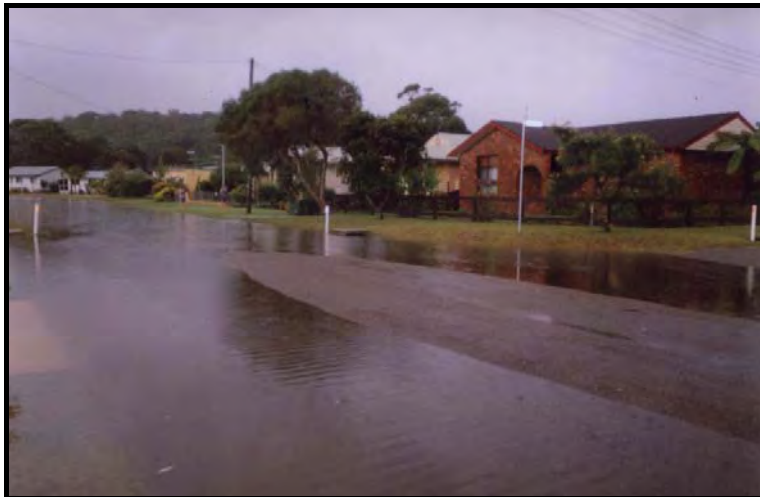
Figure 19 Thistleton Drive (cnr. Ronald Ave) - June 2005 (stormwater backing up from surcharged pipes after heavy rainfall)
