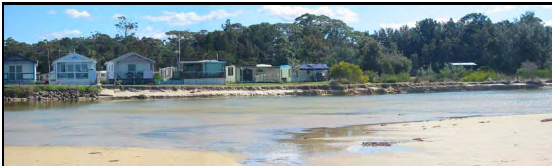
Figure 6 Dolphin Point Tourist Park showing ebb channel scour at waterline along the upstream reserve
