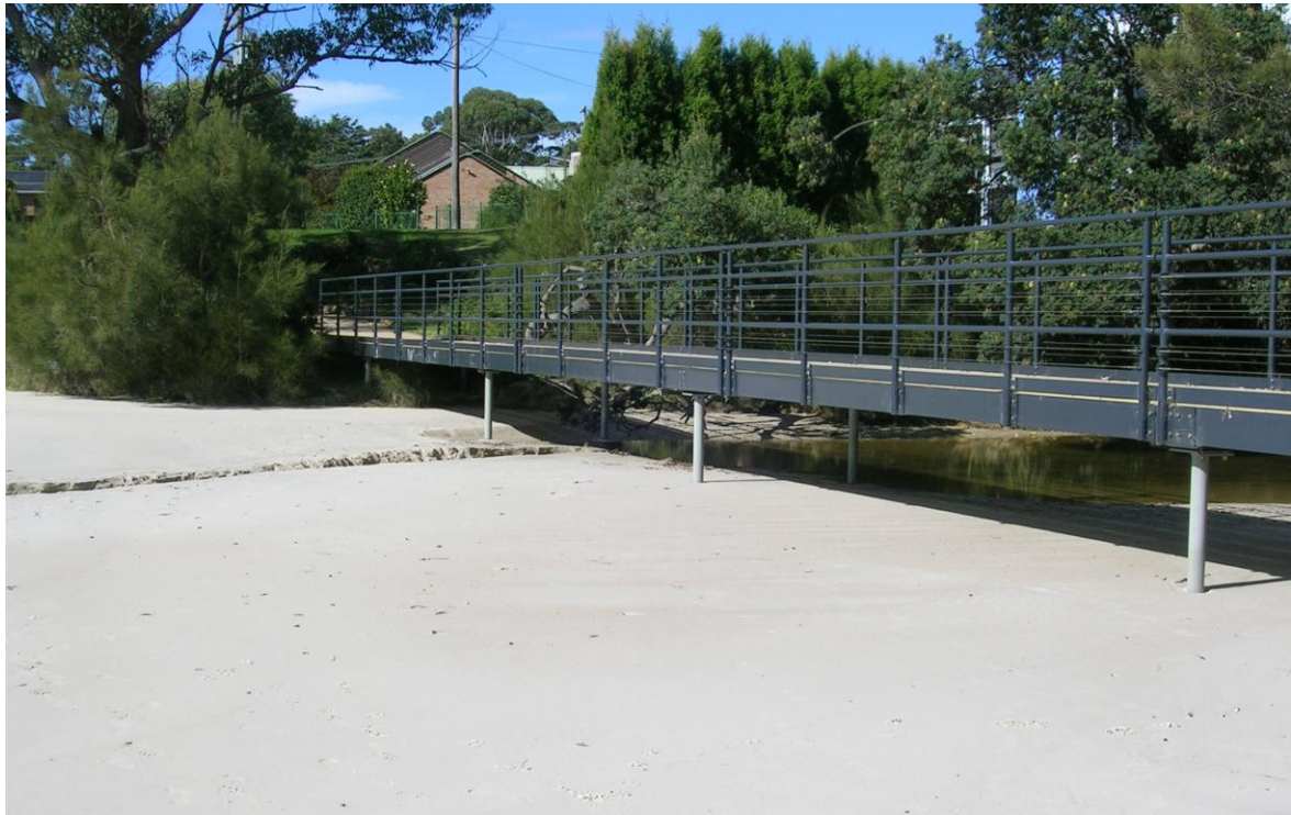
Figure 4 – An example of a recent bridge construction (west of the Holden Street Boat Ramp, Vincentia) with an approximate construction cost of $225,000.
