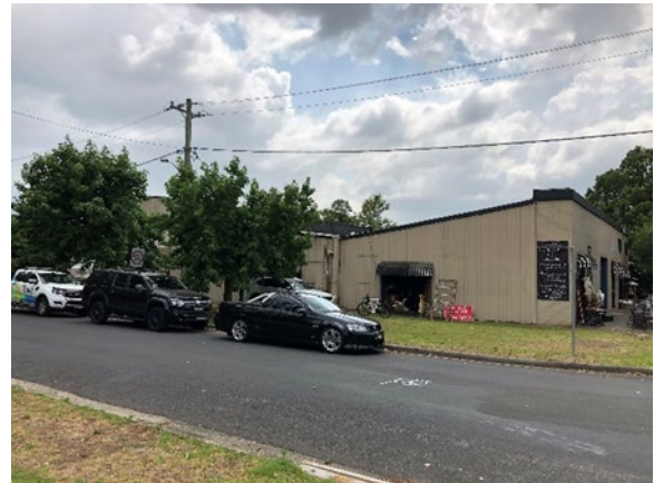
Plate 2: View of the subject land viewing north/west (*Source: MMJ Planning)
