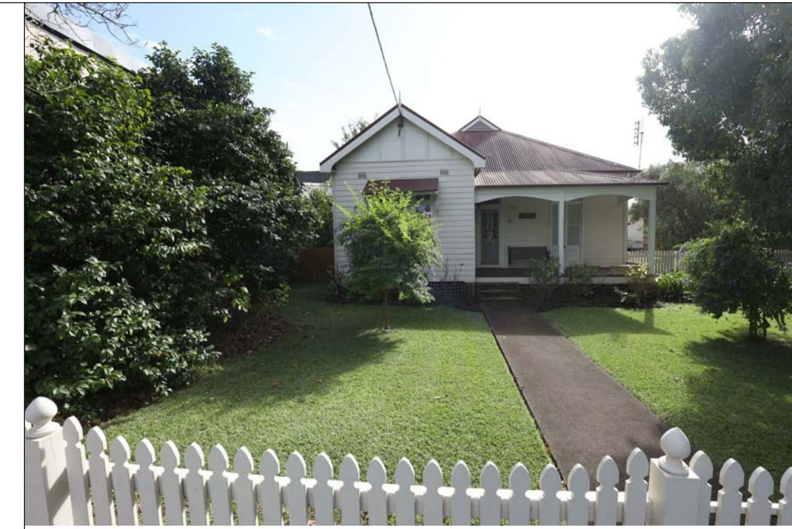
2. EARLY 1900'S EDWARDIAN HOUSES LIKE THIS ONE ARE A KEY TYPOLOGY'S WITHIN THE AREA. COMMON FEATURES INCLUDE METAL HIPPED ROOFS WITH LOW PITCH VERANDAHS. HORIZONTAL WEATHERBOARD CLADDING AND TIMBER WINDOWS ARE ALSO FEATURED.
