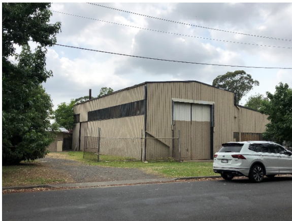
Plate 3: Existing factory sheds on site (*Source: MMJ Planning)
