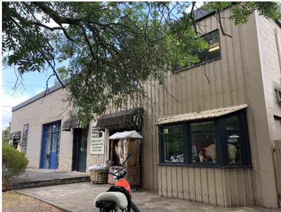
Plate 1: View of the Queen Street frontage viewing north/west (*Source: MMJ Planning)
