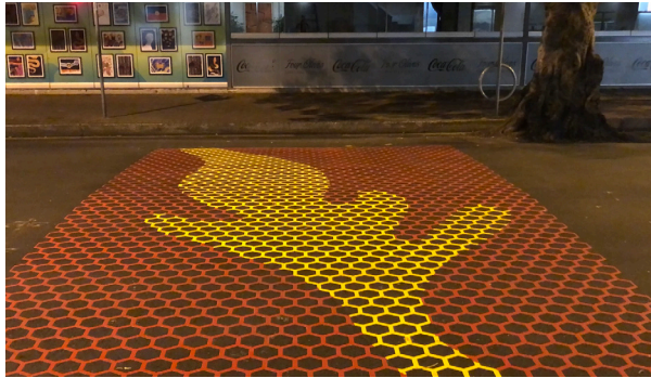
DURATHERM SURFACE FOR CARRIAGEWAY
