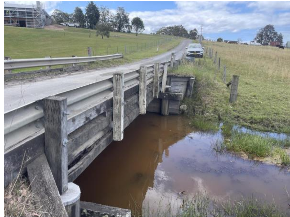
Smarts Bridge, for replacement
