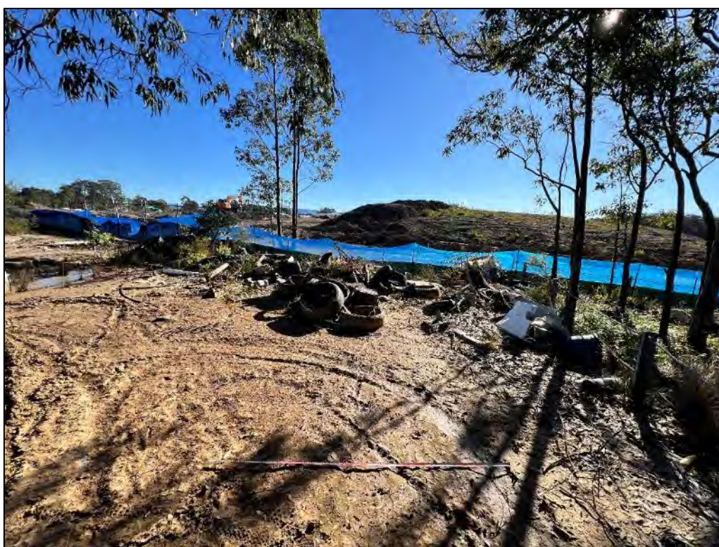
Plate 28: Dumping across the northern boundary of the site.
