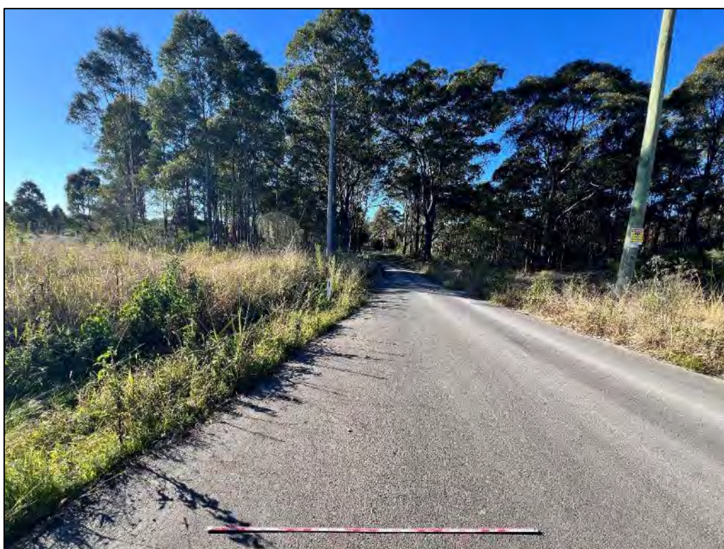
Plate 21: Looking east along Warra Warra Road and the southern boundary of the study area.
