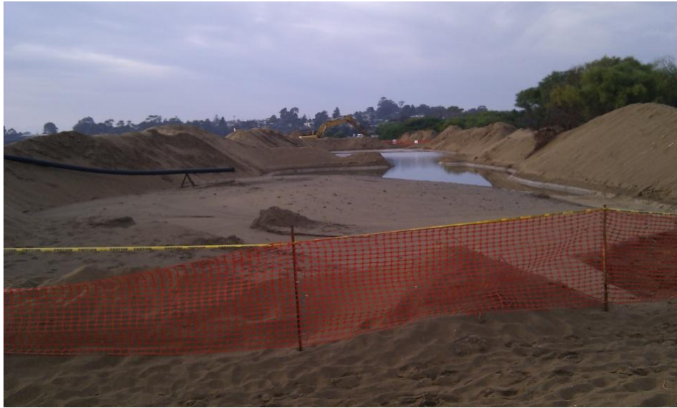
Figure 2 Dewatering bunds at Corrigan's Beach, Batemans Bay with recent dredged sand in the foreground
