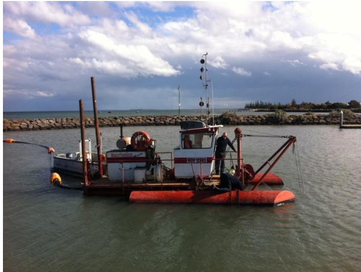
Figure 1 Small 150mm Cutter Suction Dredge
