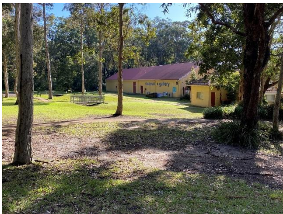
View looking north-east across drainage swale towards main entry to museum building
