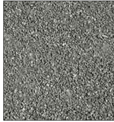
Compacted Road Base
