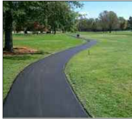
Asphaltic Concrete (Bitumen) - access roads & pathways.
