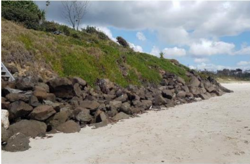
Rock Revetment at Belongil Beach
