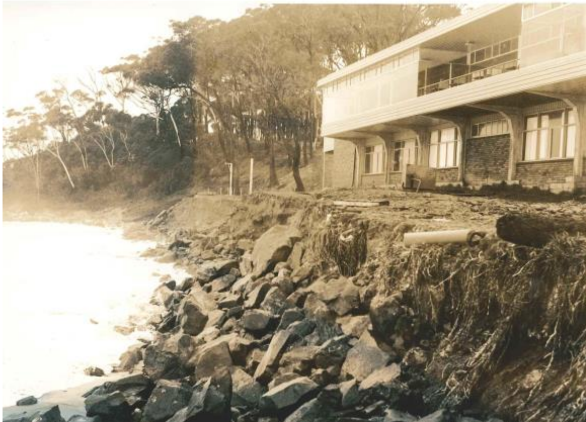
Rock protection in front of the Golf Club to counter erosion from 1974 Storm
