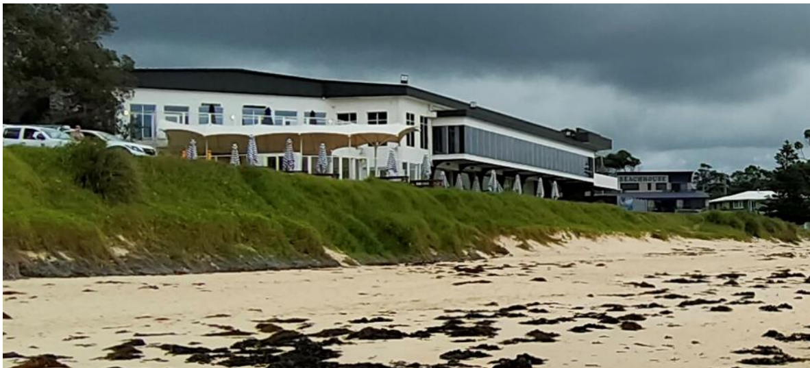
Gabion Revetment Mollymook – proposed upgrade would be buried and be of similar appearance
