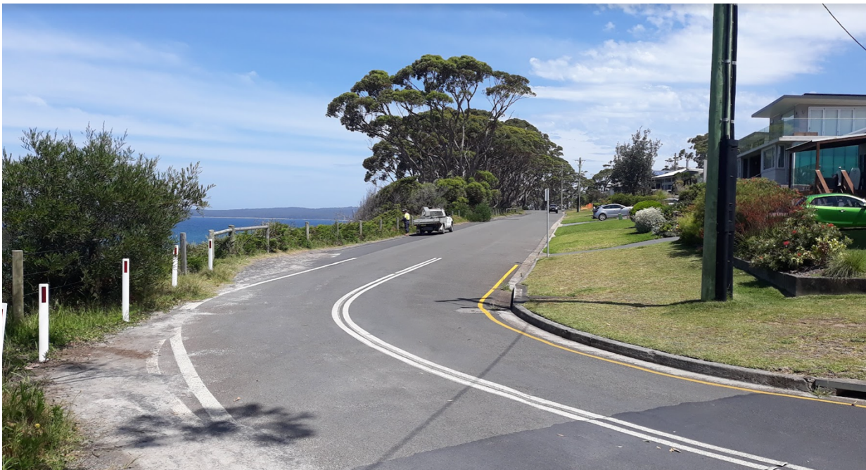
Photo 3: northern end of Cyrus Street where carparking will be formalised and footpath along the eastern edge (left-hand side) would be constructed.
