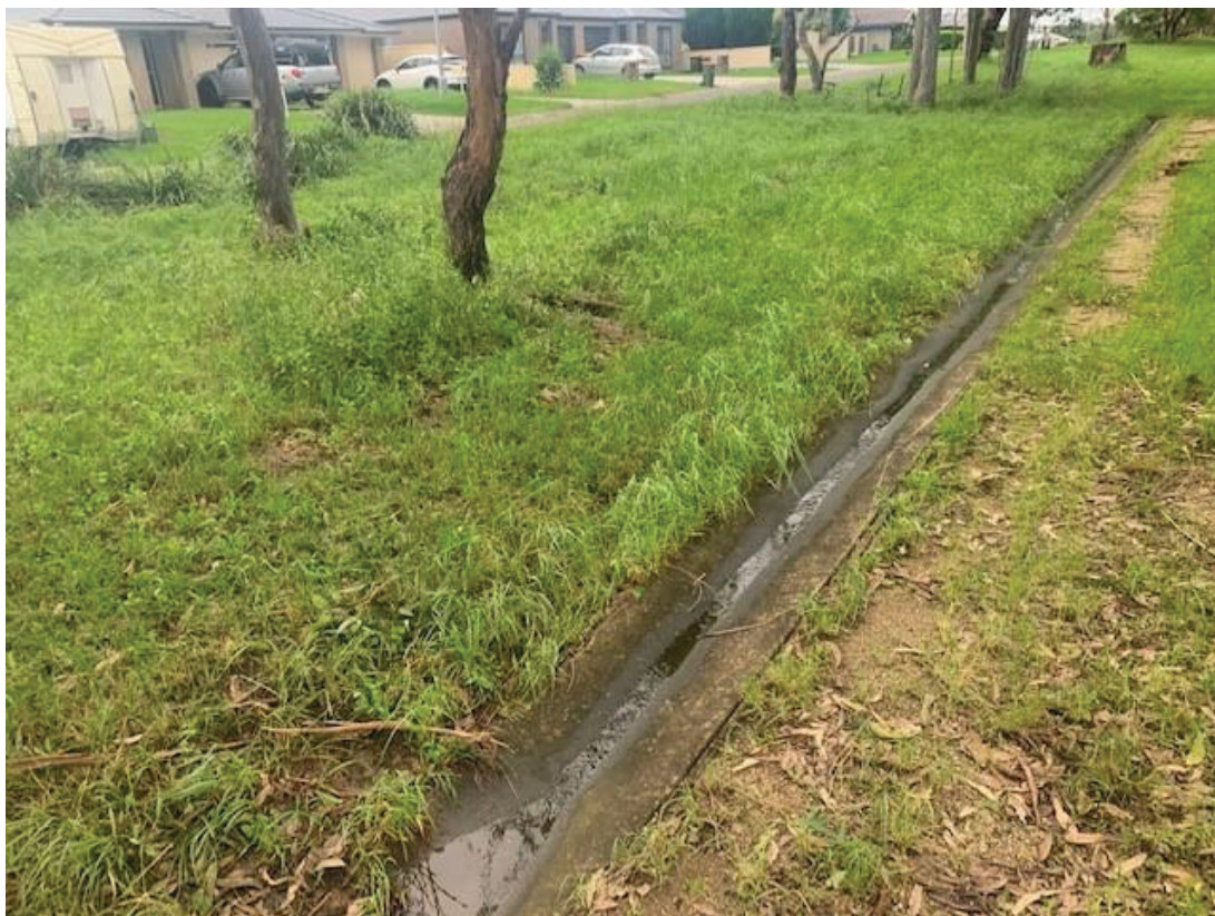
Photograph 21: Concrete drain along Garden Walk looking south-west.
