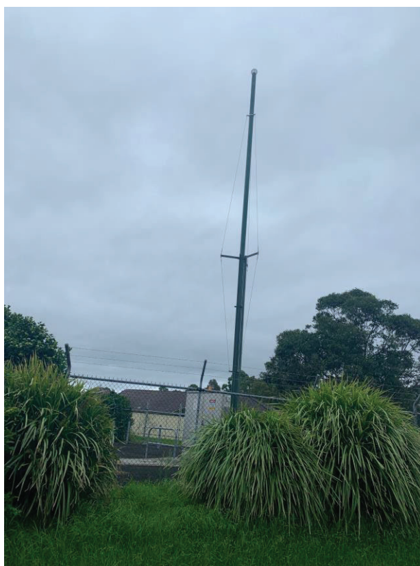
Photograph 14: Electrical storage facility at north-west corner of site looking south.
