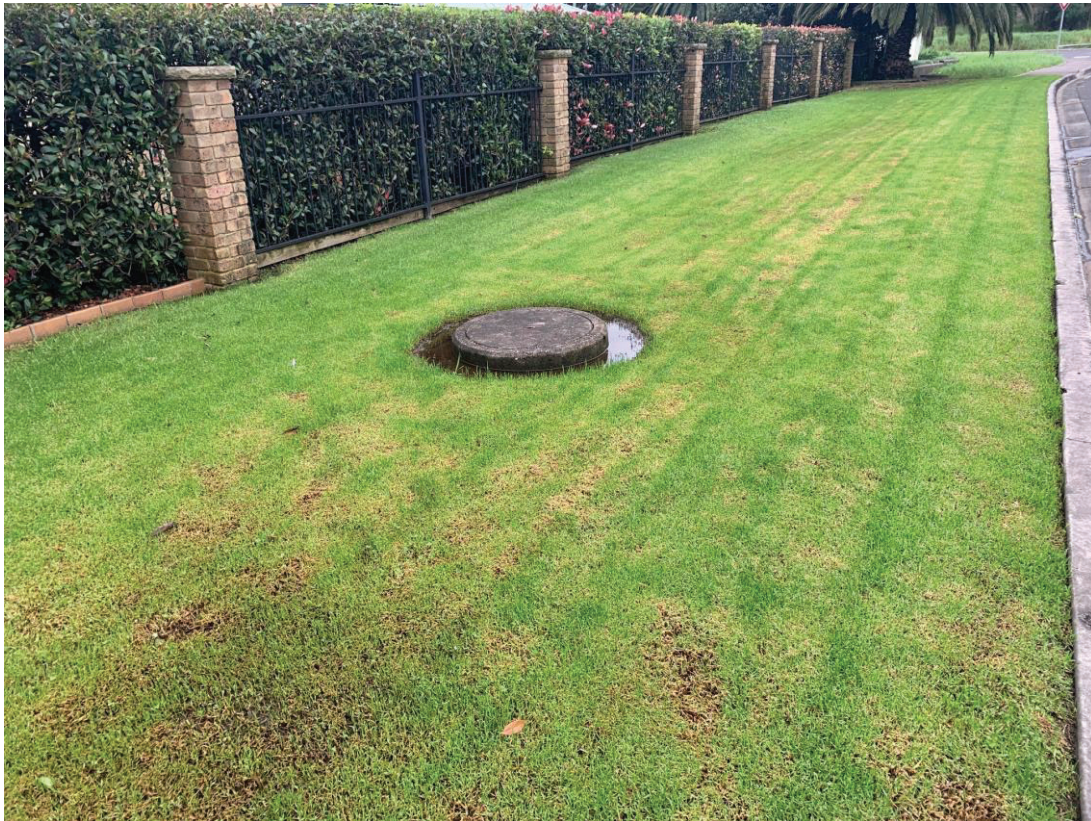
Photograph 9: Sewerage manhole along Carrington Park Drive looking east.
