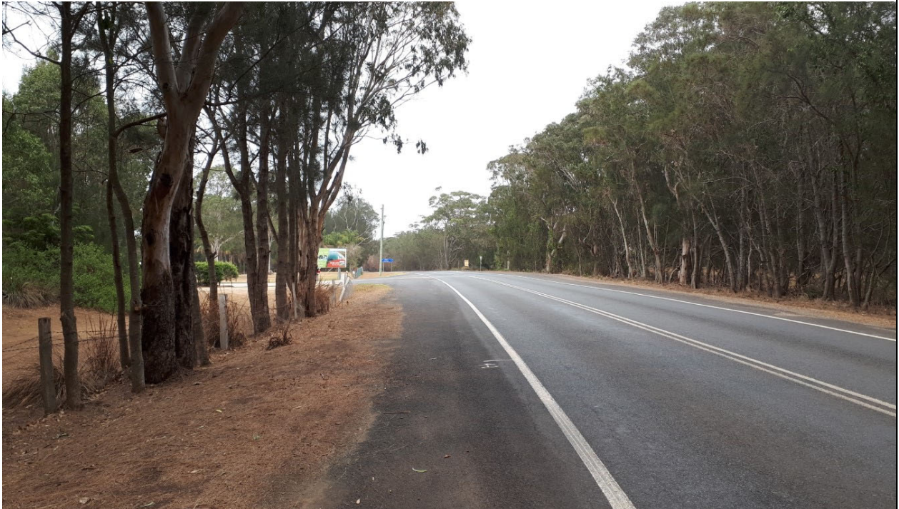
Photo 6. Southern end of Area C and Area D (cleared)
