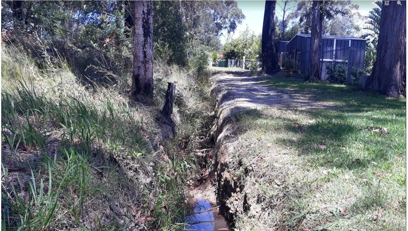
Photo 2: Existing outlet north of Sandra Street (Windermere Drive Reserve). New piped outlet to be provided with headwall and scour protection.
