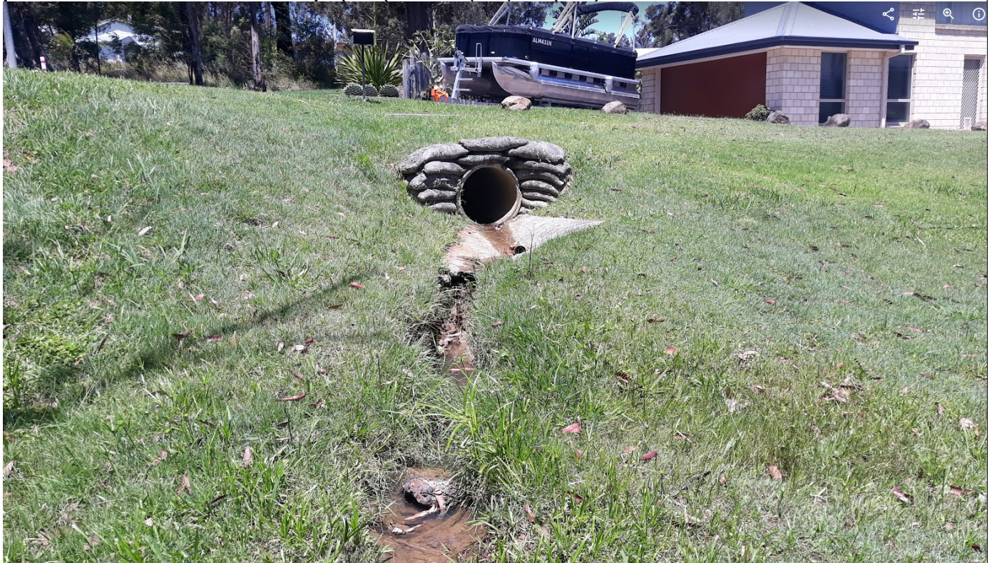
Photo 2: Existing outlet north of Sandra Street (Windermere Drive Reserve). New piped outlet to be provided with headwall and scour protection.
