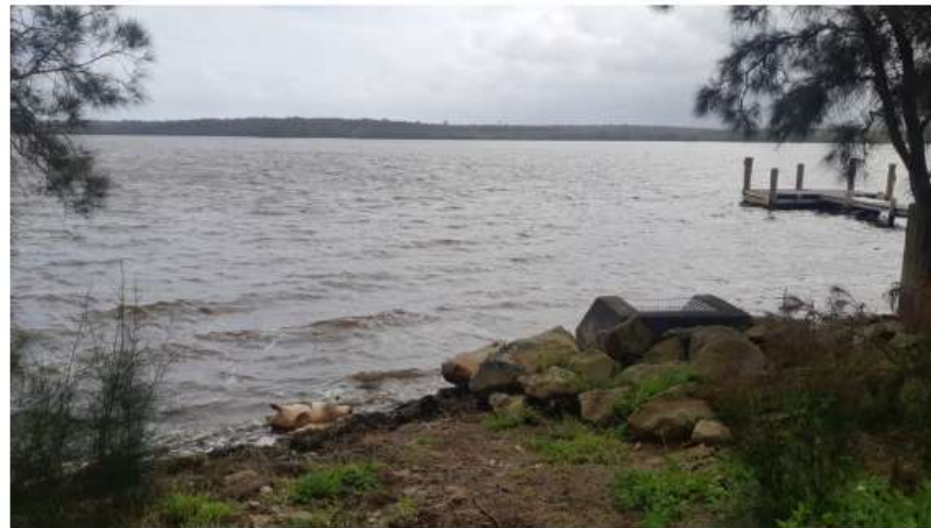
Figure 3-9 – Basin View – Mathie Street foreshore. Top – building rubble at top of bank; bottom – rock revetment protecting foreshore infrastructure.
