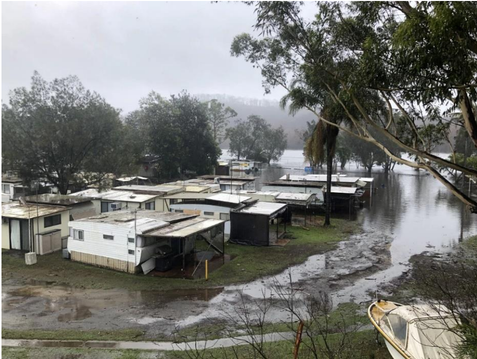
Figure 4-17: Flooding of one of the upstream caravan parks at Lake Conjola on 10 February 2020 ( www.sbs.com.au )
