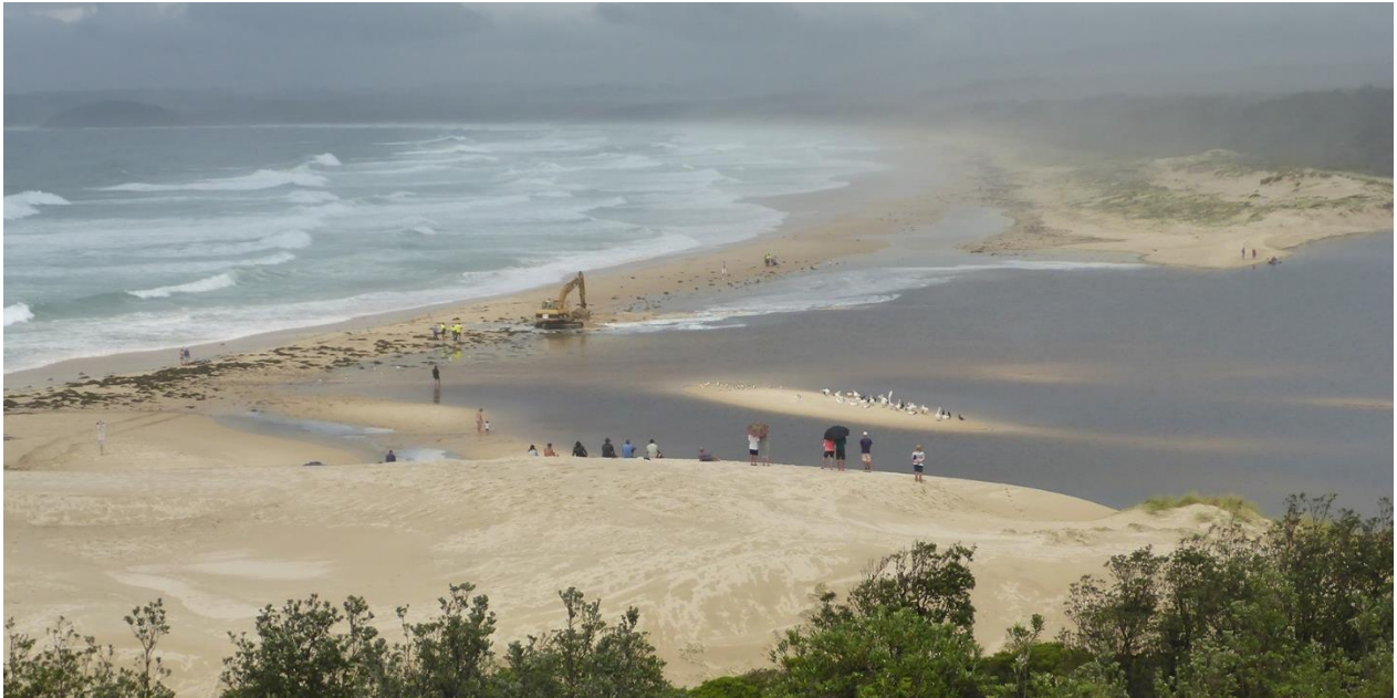
Figure 4-13: View of excavation of pilot channel in February 2020 from Cunjurong headland (source: D. Wiecek, DPE)
