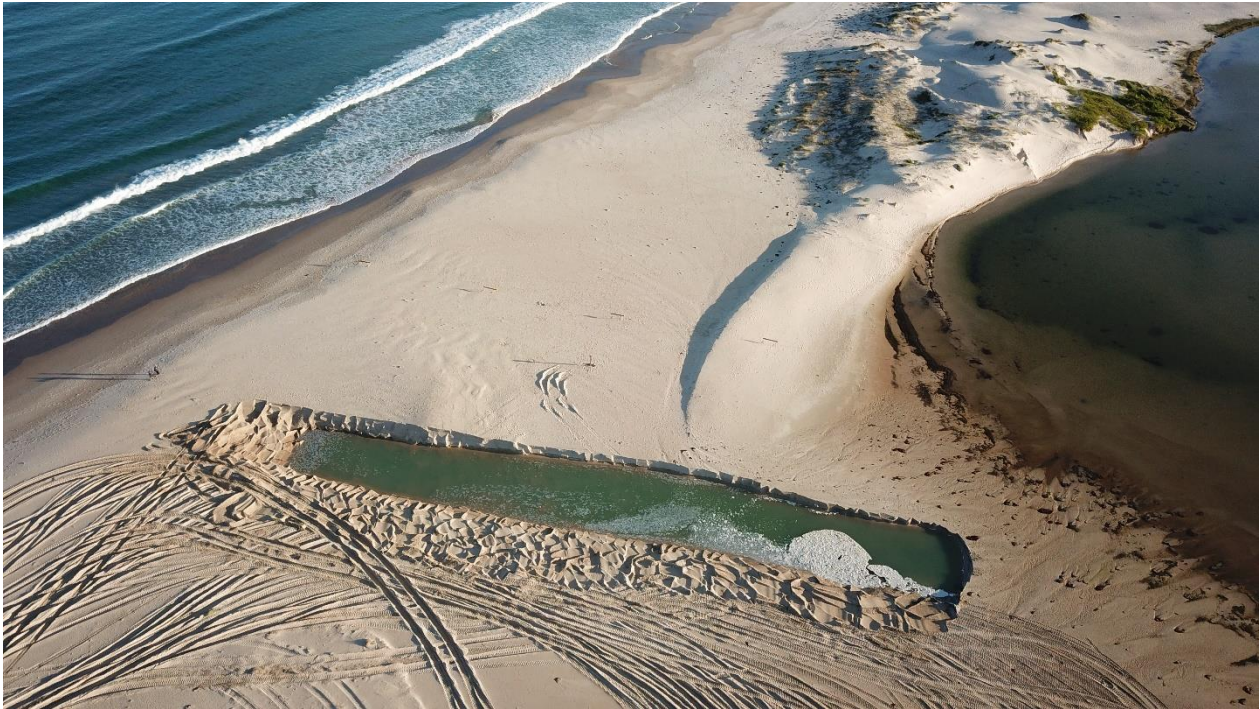
Figure 4-8: Oblique north-south aerial image - Lake Conjola mechanical entrance clearance works - June 2019 (source: Shoalhaven City Council)
