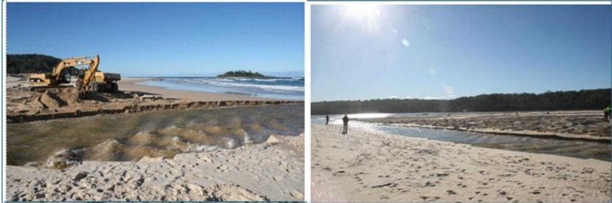
Figure 4-10: Mechanical opening of Lake Conjola entrance near high tide around 10am 19 June 2019, with water observed flowing out of the lake from around 1:45pm 19 June 2019 (source: D. Wiecek, DPE)
