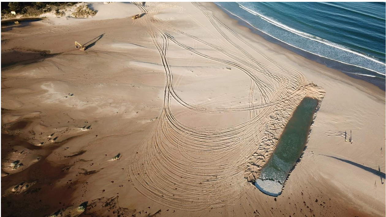
Figure 4-9: Oblique west-east aerial image - Lake Conjola mechanical entrance clearance works - June 2019 (source: Shoalhaven City Council)
