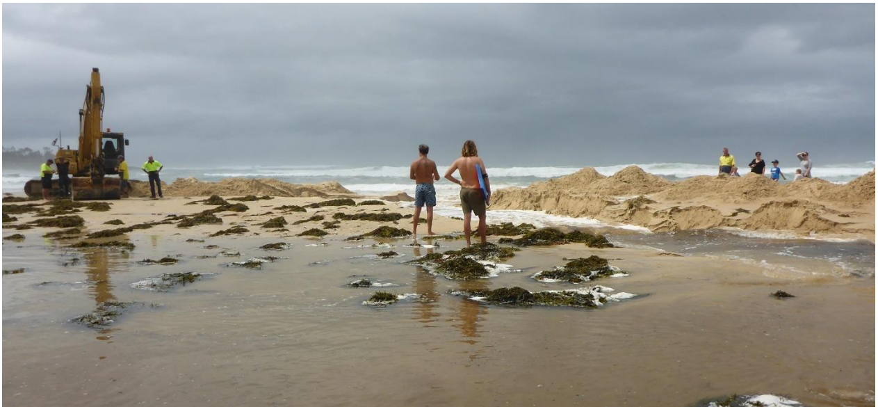
Figure 4-14: Close up view of excavated pilot channel in February 2020 with outflow occurring (source: D. Wiecek, DPE)
