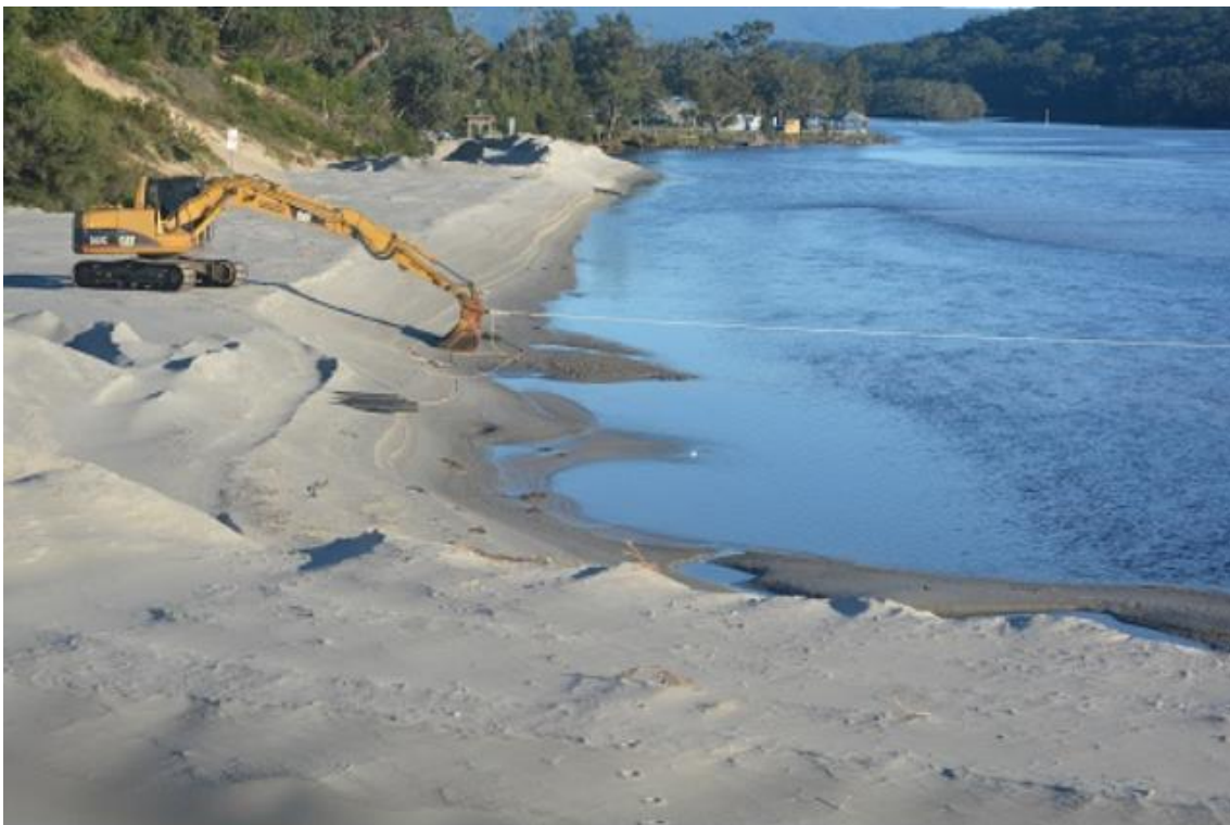
Figure 4-22: View of the sand placement area along the southern shoreline
