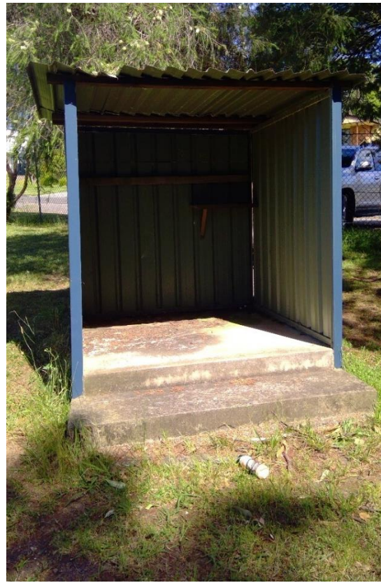
Plate 2: Existing shed infrastructure within the dog off-leash access area.
