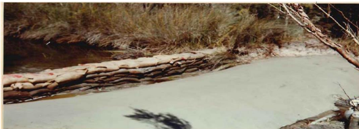
Figure 8-15: The weir being installed at the entrance of Pattimores Lagoon in 1982 by Shoalhaven City Council (Clarke, 2012)
