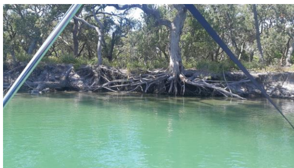
Continuing erosion of sandy foreshore, downstream Little Manly, Sussex Inlet
