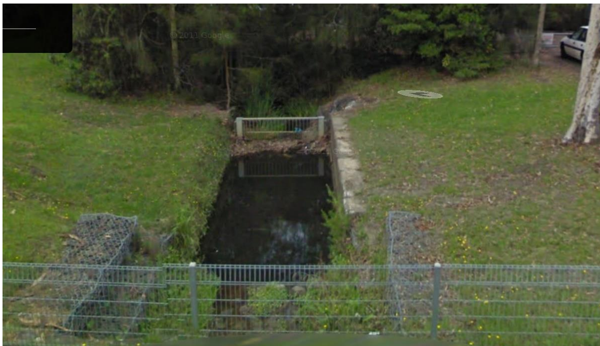
Figure 6-10 – Example trash rack at Sanctuary Point (Google Maps street view)
