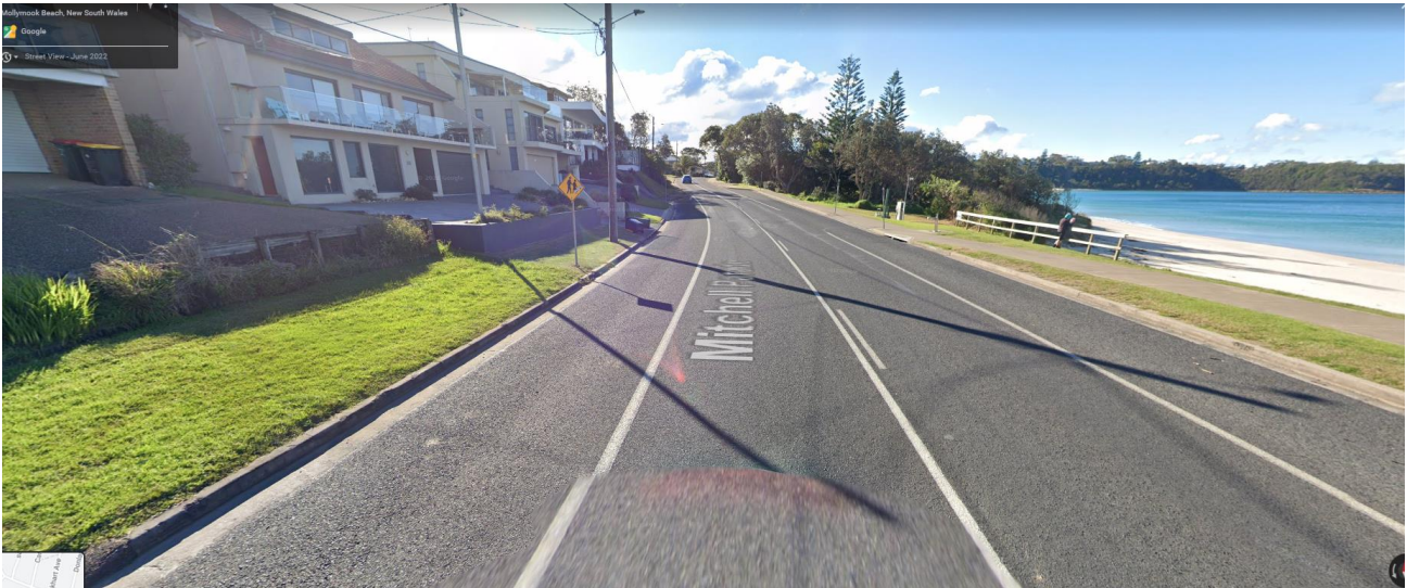
Figure 5-1 Mitchell Parade at the proposed works site (image source: Google StreetView)
