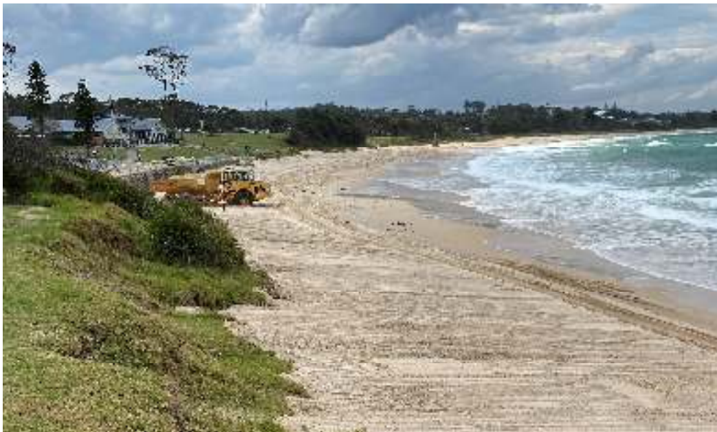
Figure 5-4 Mollymook Beach Erosion and subsequent beach scraping in mid-2020. Image source: SCC
