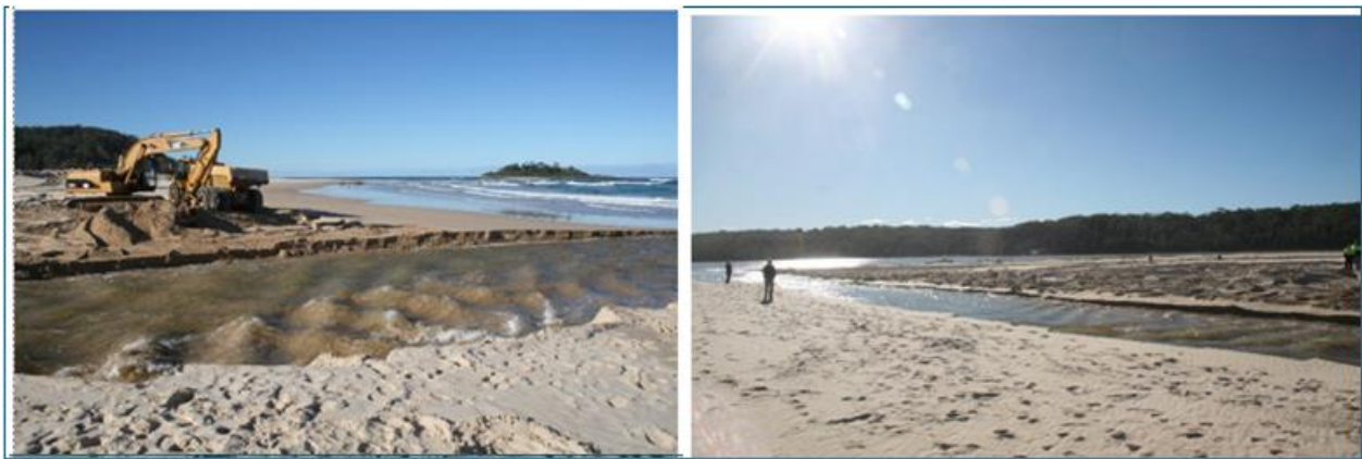
Figure 5-13: Mechanical opening of Lake Conjola entrance in June 2019 (source: D. Wiecek, DCCEEW)
