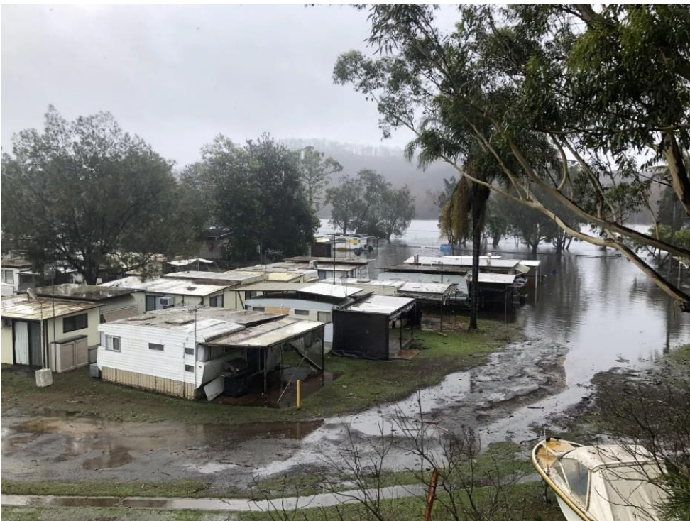
Figure 5-2: Flooding of one of the upstream caravan parks at Lake Conjola on 10 February 2020 ( www.sbs.com.au )
