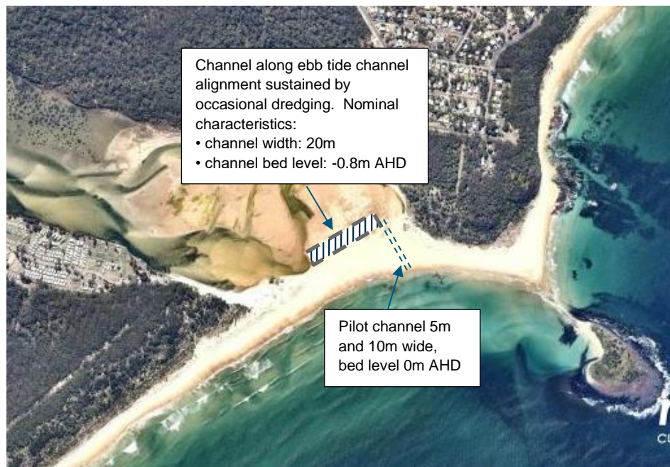
Figure 4-1 Diagram summarising concept for Category 3 entrance management options – air photo date 14 September 2018 (Figure 5-4 from RHDHV Report C, March 2023)
