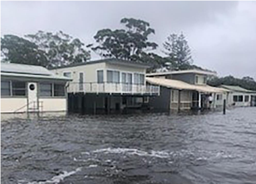
Figure 5-1: Flooding of houses in Lake Conjola Village on 10 February 2020 (courtesy of Ms Kristen Bird)
