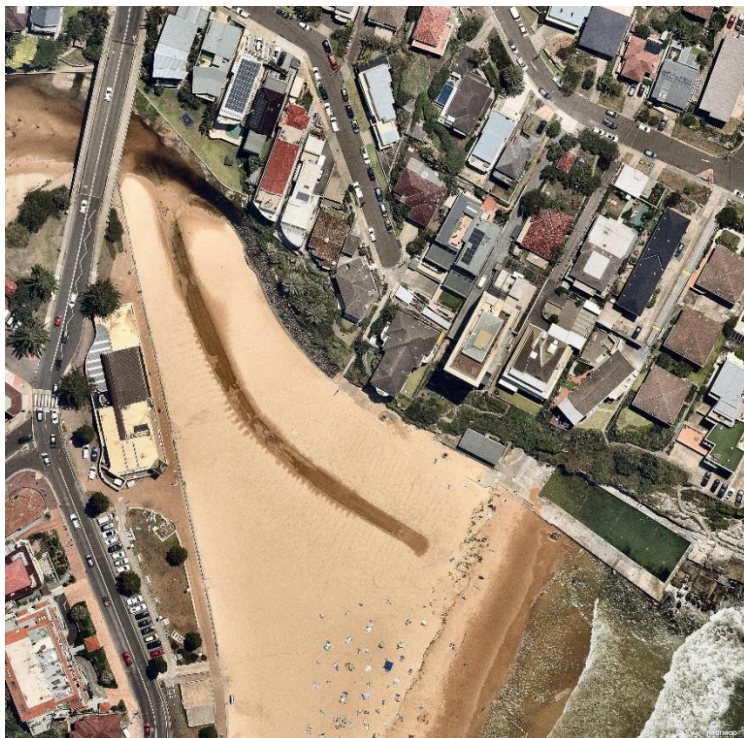
Figure 5-15: Example dry notch maintained at the entrance to Manly Lagoon, Queenscliff Beach (January 2020)
