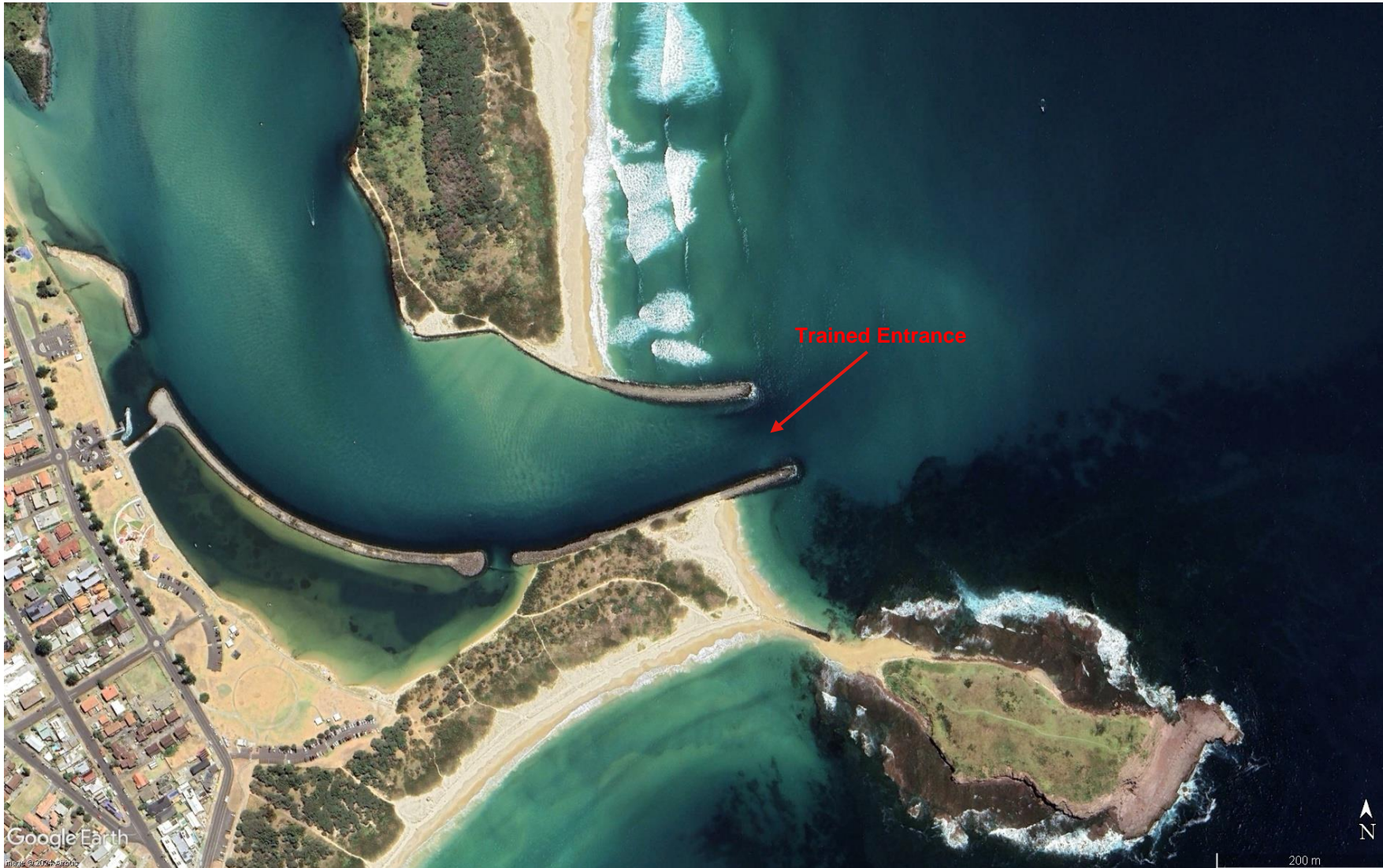
Figure 3-9: Lake Illawarra entrance training walls (source: Google Earth Pro dated 23 December 2022)
