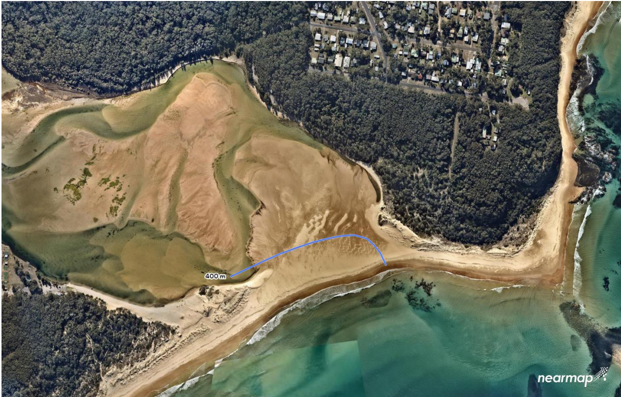
Figure 5-5: Aerial photograph showing an example of the Storm Washover Entrance State and indicative pilot channel alignment from northern spit zone shown in blue linework (source: Nearmap, dated 15 July 2018)
