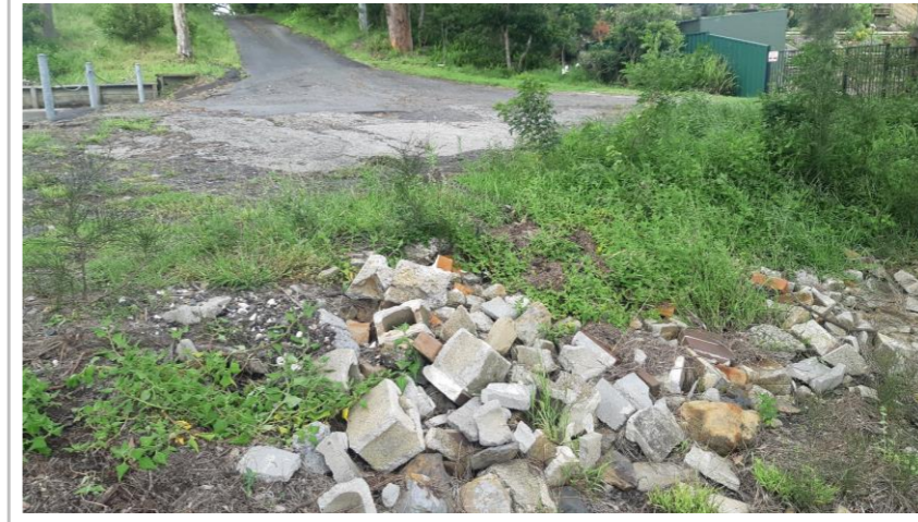
Building rubble on upper section of bank at Mathie St Site Ref BV03
