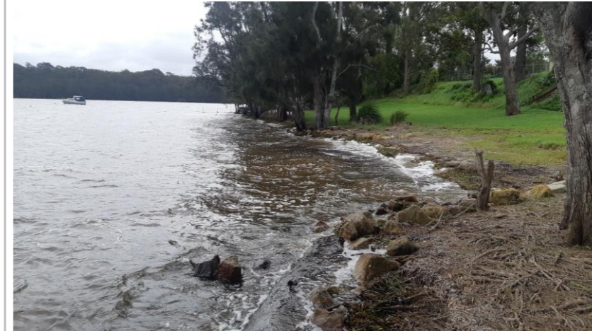
Looking west from Basin Road Jetty Site Ref STB02
