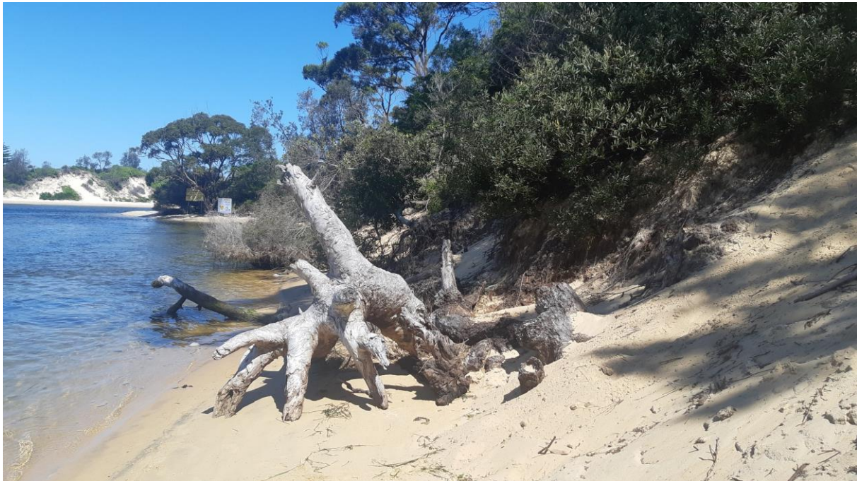
Figure 4-11 – The Haven, southern end, looking south. Note erosion occurring due to slope instability and wave action at the toe of the slope (1 December 2021). Site reference H03.
