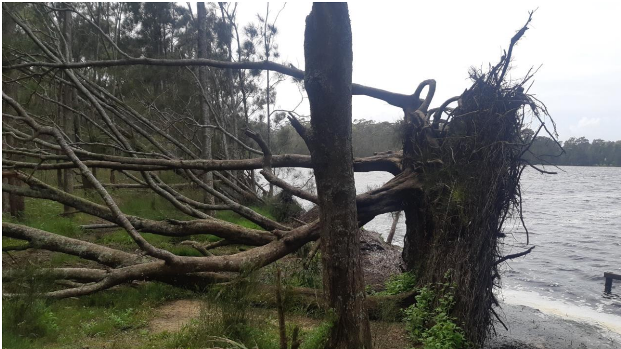
Figure 3-34 – Old Erowal Bay foreshore. Top – at Prentice Avenue Reserve, bottom - looking east along foreshore from reserve area. Note undercutting of casuarinas leaving them vulnerable to toppling and loss of root ball leading to soil loss from the bank (28 November 2021). Site reference OEB01.
