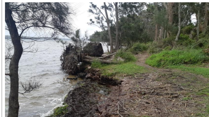
Foreshore erosion at The Basin Walk, Macleans Point Site Ref MP01
