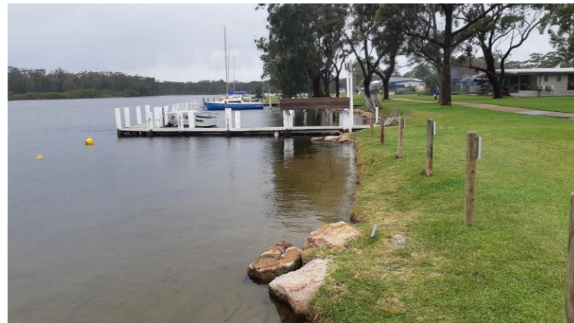
Rock fillets and moorings catering to holiday accommodation Site Ref S004
