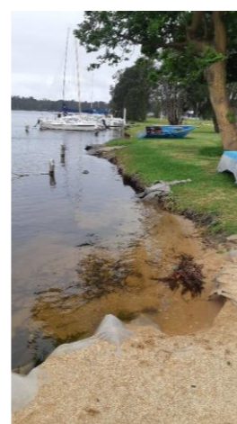
Sandy foreshore with imported sand and geotextile Site Ref S004
