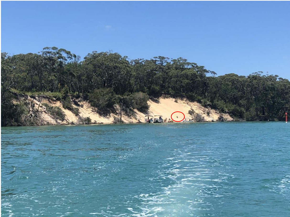
Figure 4-20 – Area at Little Manly is popular for recreation, unstable slope could be a safety hazard (7 December 2021). Note slope being used for sand-boarding. Site reference S011.
