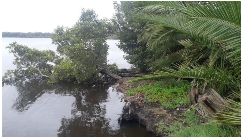
Erosion at entrance to Badgee Lagoon, downstream River Road Bridge Site Ref S003
