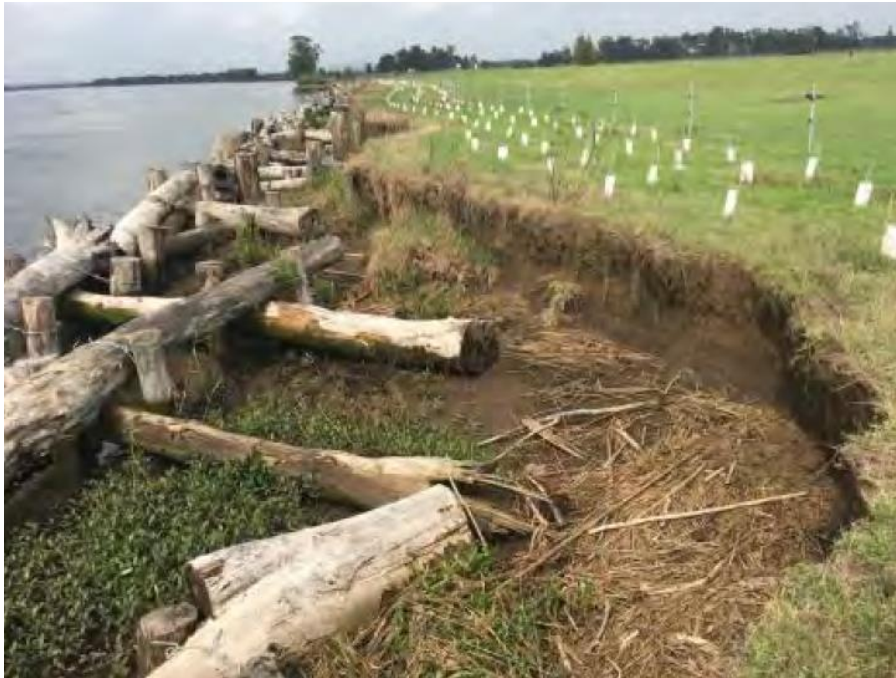
Figure 3-5 – Application of large woody debris at Hunter River, NSW. (Hydrosphere Consulting, 2020).
