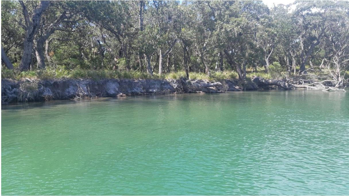
Figure 4-19 – Active bank erosion downstream of Little Manly (7 December 2021) Site reference S011.
