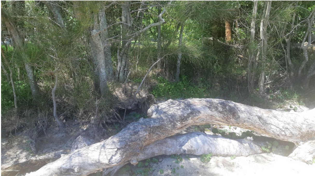
Figure 5-8 – Minor bank erosion at upper bank at Swan Lake Ski Beach (top, site reference SW05), Dyball Reserve (bottom, site reference SW02), 1 December 2021
