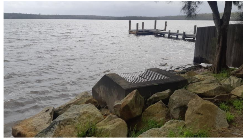
Rock revetment protecting sewer infrastructure at Mathie St Site Ref BV03
