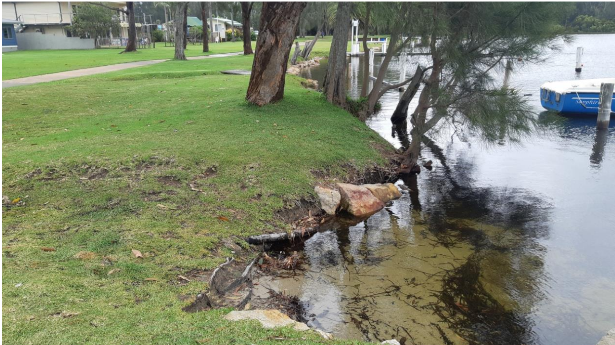
Figure 4-30 – Foreshore protection works at Sussex Inlet, upstream of Nielson Lane boat ramp, looking west (27 November 2021). Site reference S004.
