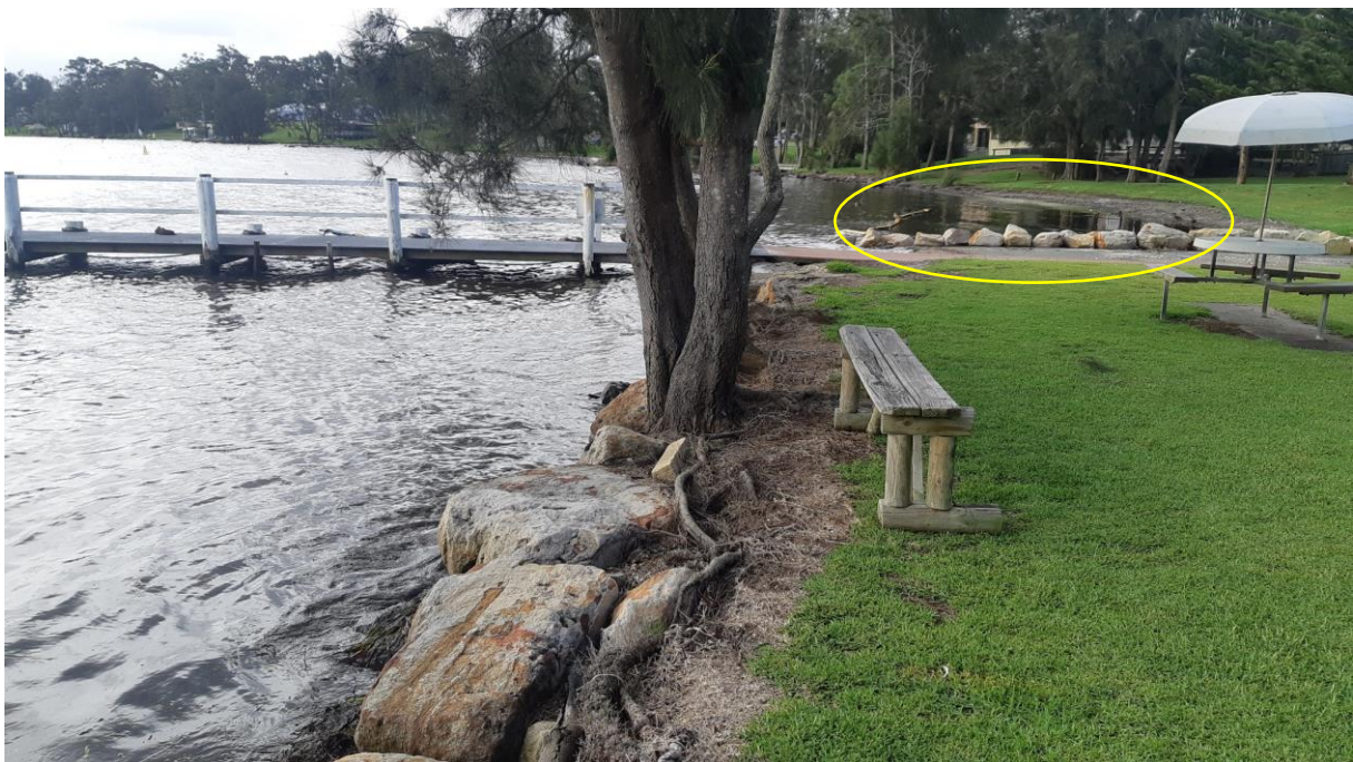
Figure 3-21 – Aloha Caravan Park frontage showing foreshore erosion protection works, jetty and beach area in background. A litter boom is installed in front of a stormwater outlet in the area circled in the image (28 November 2021). Site reference STB01.
