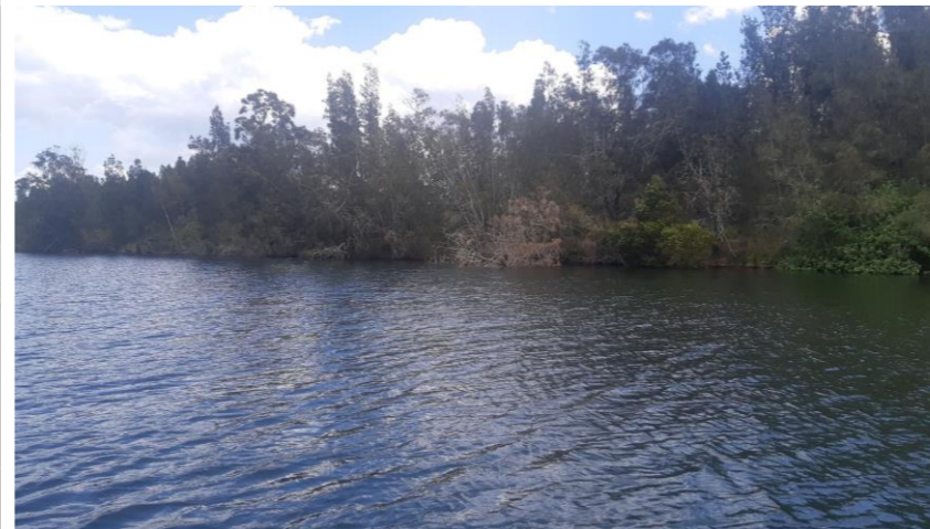
Ralph Lucas Waterway undermining of trees Site Ref S010
