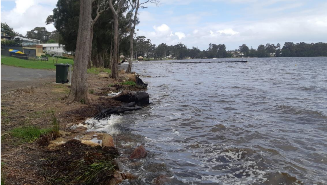
Figure 3-22 – Minor rock works installed at The Basin Road foreshore public access area (28 November 2021). Site reference STB02.
