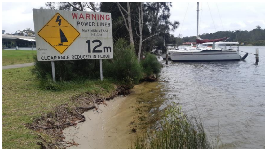
Eroded foreshore, Jacob Elimoos Reserve Site Ref S007
