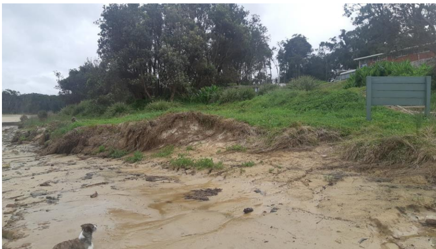
Figure 6-2 – Erosion looking upstream from Berrara Creek beach access (1 December 2021). Site reference BC01.
