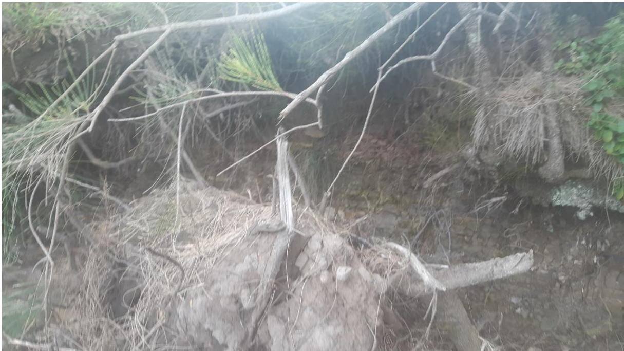
Figure 6-5 – Bank erosion showing sections of bank detaching from foreshore and high vertical erosion scarp (1 December 2021). Site reference BC03.
