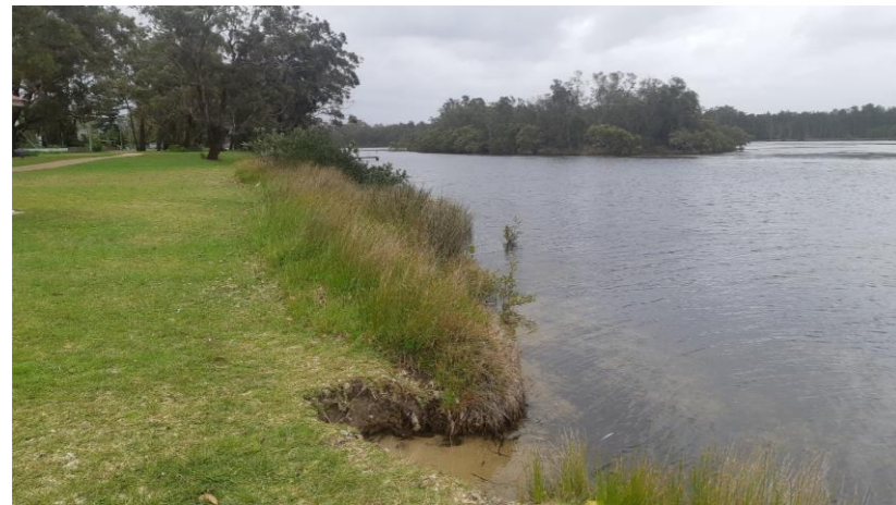
Minor erosion upstream from Sussex Marine Centre Site Ref S005
