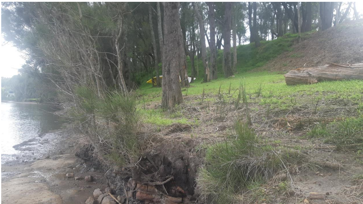
Figure 6-7 – Minor erosion and vertical scarp at Berrara Waters foreshore with use of adhoc building rubble to contain erosion (1 December 2021). Site reference BC04.
