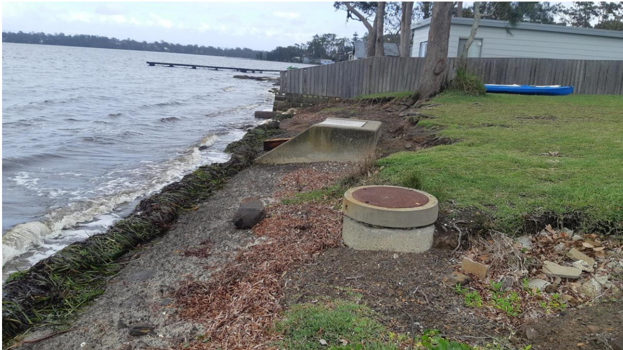
Figure 3-37 – Erowal Bay foreshore at Wharf Road (28 November 2021). Site reference EB01.
