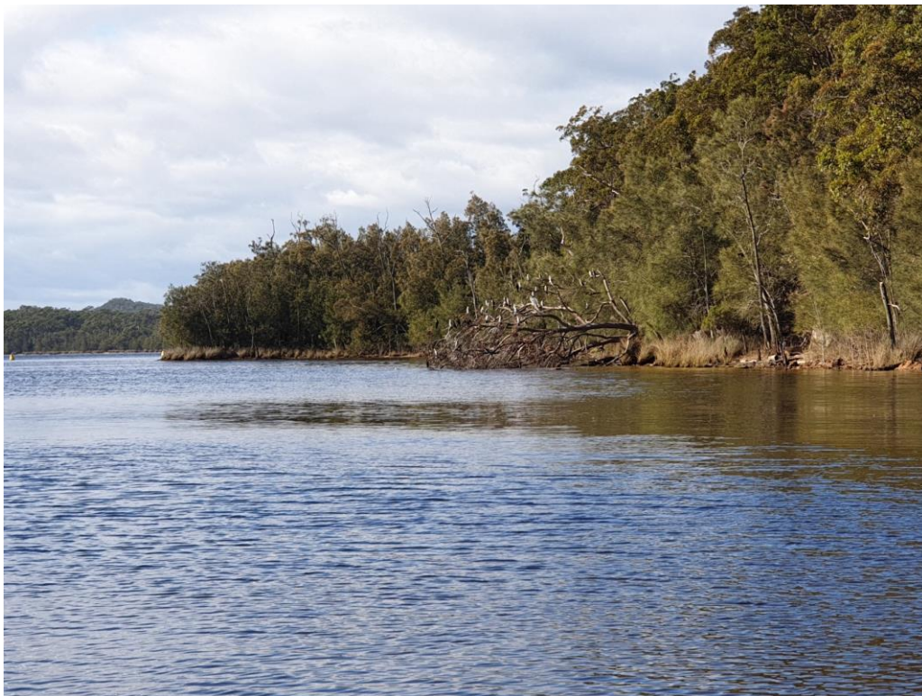
Figure 5-12 – Dead trees at risk of toppling causing destabilisation of bank. Note that these trees are used as roosting habitat for birds (17 June 2022). Top: site reference SW04, bottom: site reference SW08.
