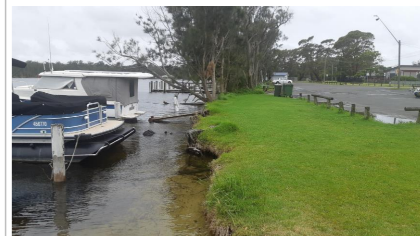
Eroded foreshore behind moored boats, upstream from Nielson Lane Boat Ramp Site Ref S004
