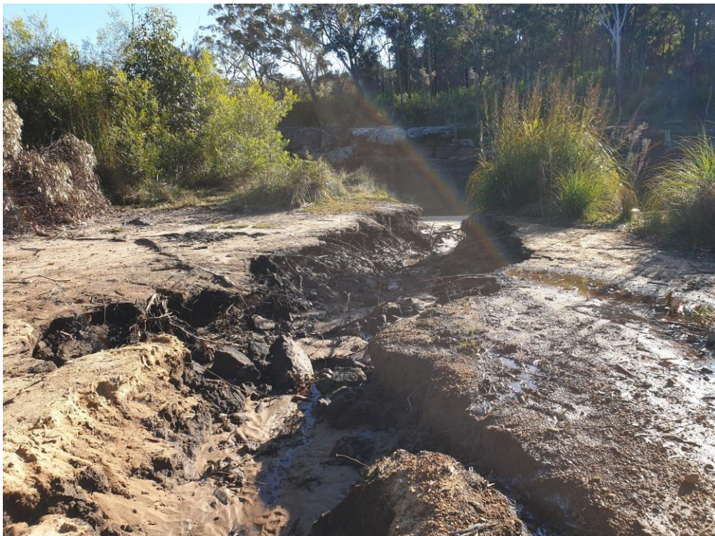
Figure 6-11 – Erosion at BC07, opposite Fishermans Rock, 17 June 2022. Site reference BC07.
