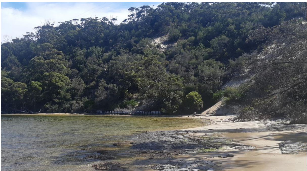
Figure 4-5 – Timber toe protection wall damaged due to overturning, caused by high earth pressures (detail on top) (1 December 2021). Site reference H05.
