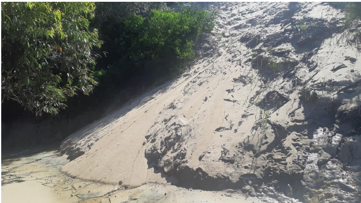
Figure 4-7 – Evidence of dune slumping caused by slope instability (1 December 2021). Site reference H05.
