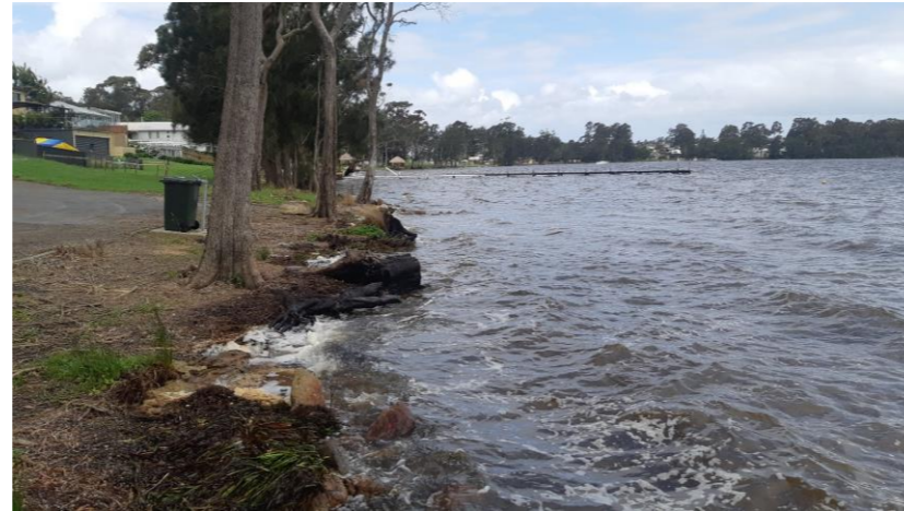
Basin Road, near Basin Road Jetty Site Ref STB02
