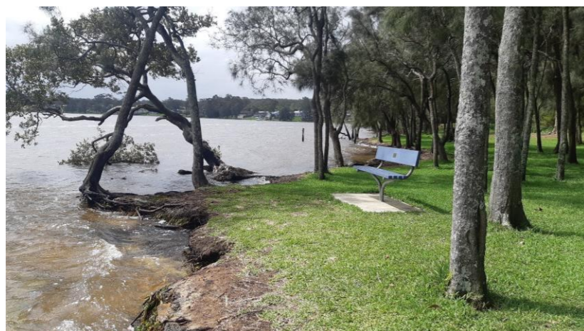
Mangrove being undermined, Blackett Reserve Site Ref STB01
