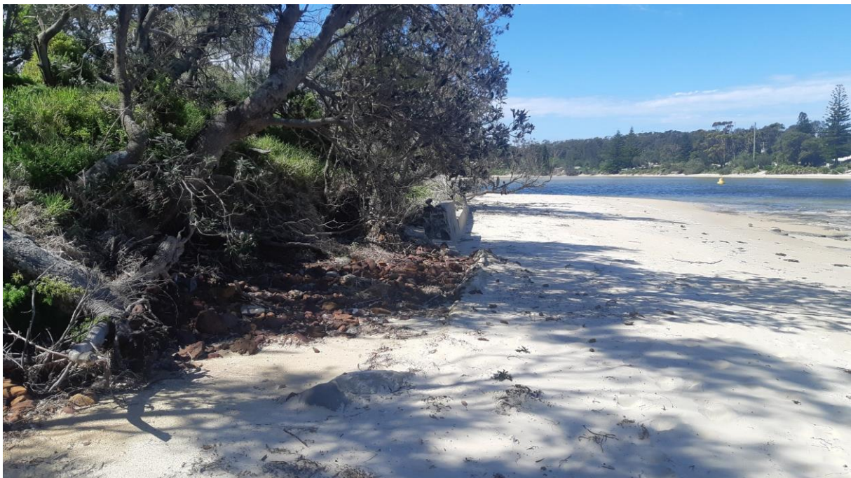
Figure 4-3 – Erosion at northern end of Croppers foreshore (H04), caused by edge effect from concrete seawall and the site exposure to ocean waves through the entrance (1 December 2021)
