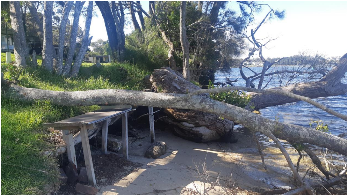
Figure 4-15 – Top: Alamein foreshore at Sussex Inlet, looking north. Bottom: detail of eroded area showing undercutting of slope (1 December 2021). Site reference S012.
