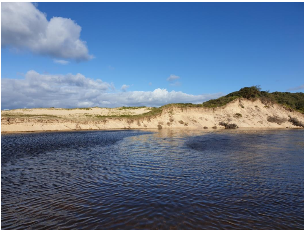
Figure 5-7 – Erosion occurring at “The Gap”, caused by seaward migration of inlet channel bend toward relict beach dunes. Note evidence of wave overtopping of the beach berm at this location (top), 17 June 2022. Site reference SW03.
