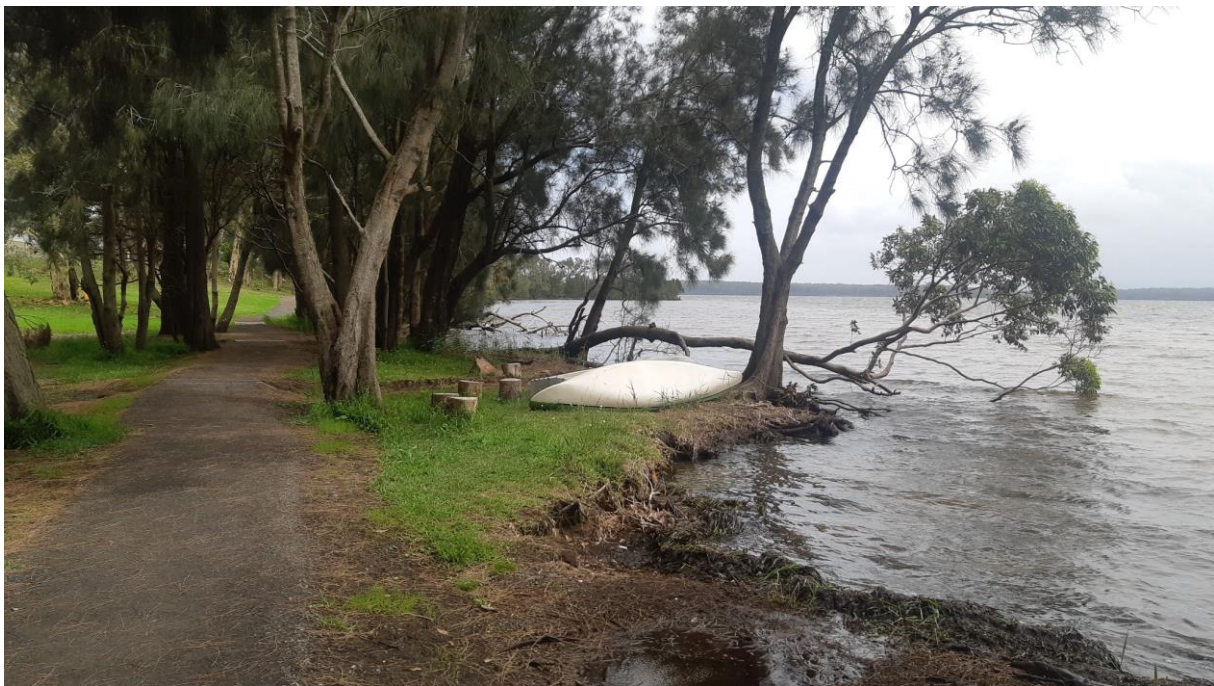
Figure 3-27 – Erosion at Lorilyn Avenue. Note adhoc storage of kayaks on the foreshore (28 November 2021). Site reference LAW01.
