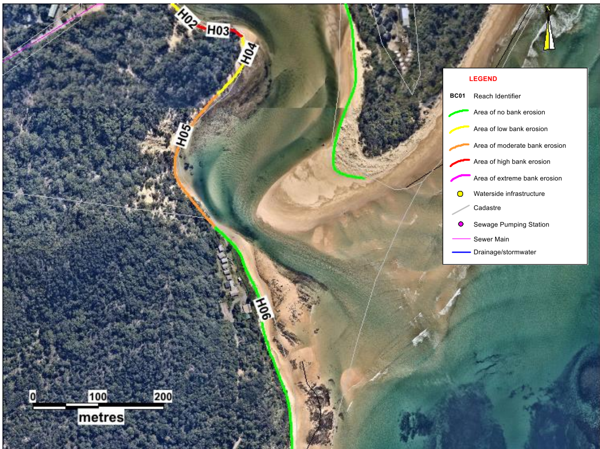
Figure 4-2 – Detail of H05 site at Croppers Cabins assessed as having erosion of moderate severity
