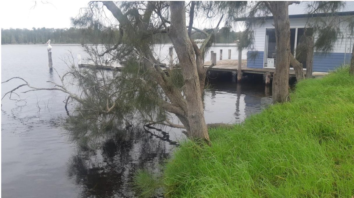
Figure 4-23 – Undermining of trees and instability due to weeds, just east of Neilson boat ramp (27 November 2021). Site reference S005.
