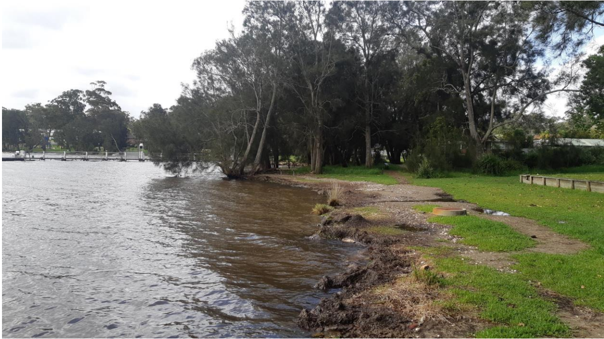
Figure 3-20 – Blackett Reserve showing active erosion and sewer infrastructure in the erosion zone (28 November 2021). Site reference STB01.
