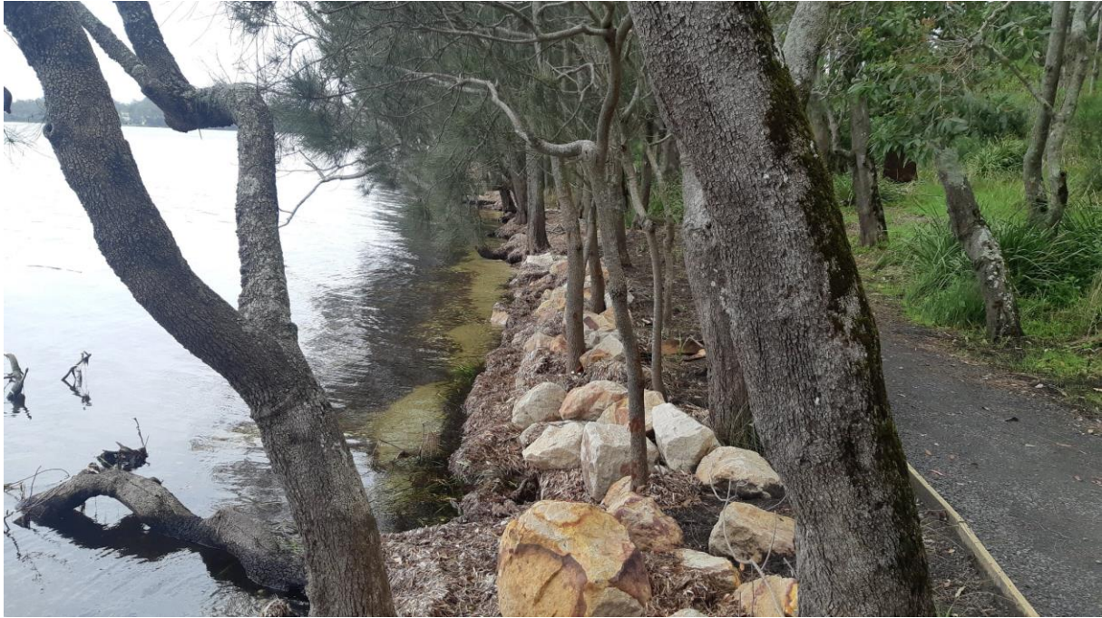
Figure 3-29 – Use of rock fillets to protect casuarina roots from undermining and provide erosion protection to Basin Track (northern end of Macleans Point, 28 November 2021). Site reference MP02.
