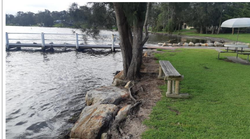
Blackett Reserve near Aloha caravan park, showing rock protection at eroding foreshore Site Ref STB01
