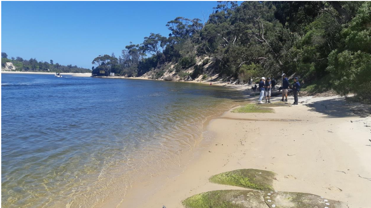
Figure 4-10 – Foreshore at The Haven, looking south. Note use of geotextile groynes combined with sand nourishment undertaken in 2017 which has protected the toe of the slope from erosion, pushed the navigation channel away from the eroding slope and improved access and amenity (1 December 2021). Site reference H02.
