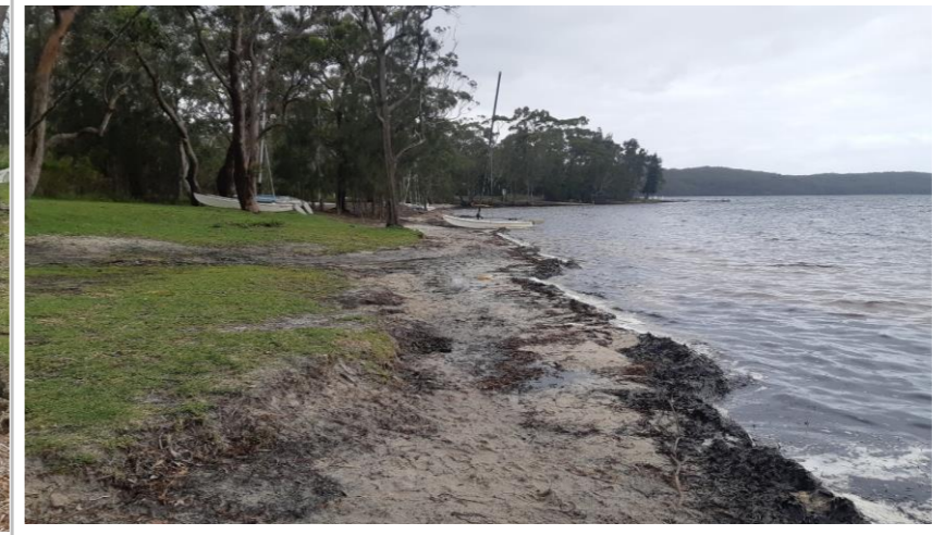
Minor erosion at Wrights Beach Site Ref WB01
