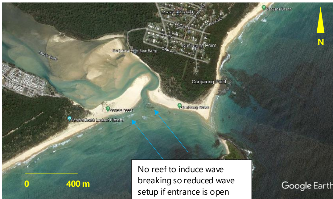
Figure 2-7 - Sand blocked entrance in front of Lake Conjola
