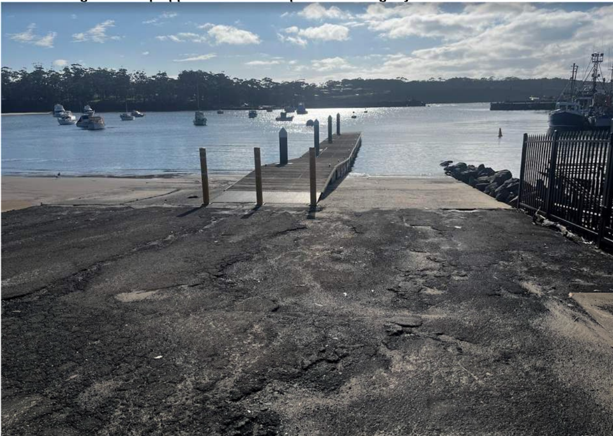
Photo 4. Existing boat ramp approaches to be replaced and slightly raised
