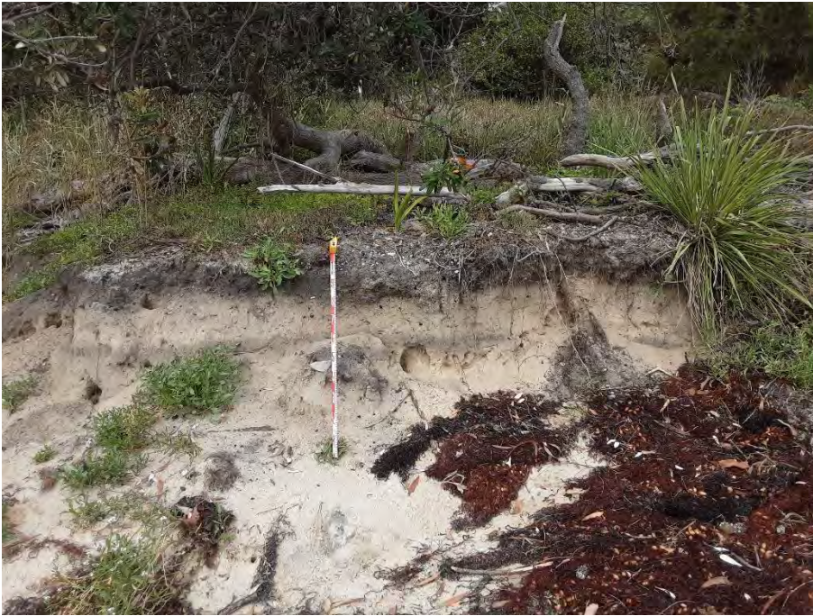
Photo 13 Disturbances caused by coastal erosion, facing west, scale 1 metre
