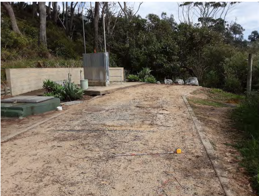
Photo 14 Disturbances from construction of water treatment station, facing south, scale 1 metre
