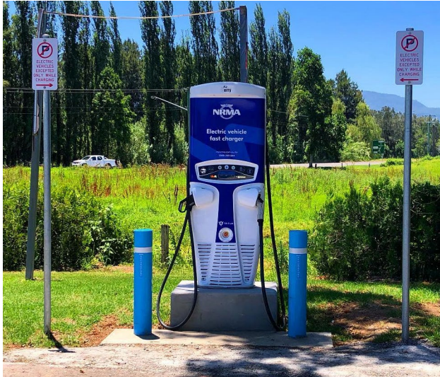
Figure 16. Electric Vehicle (EV) 50 kW DC fast charging station installed by the NRMA at the Berry Bowling Club in early 2019 (left) and 6 Tesla Superchargers installed at Silos Estate near Berry in mid-2019 (right).
