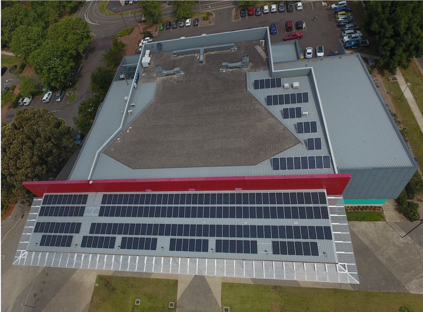
The rooftop of the Shoalhaven Entertainment Centre in Nowra showing the 81kW solar PV installation (200 solar panels) completed in Oct 2019.
