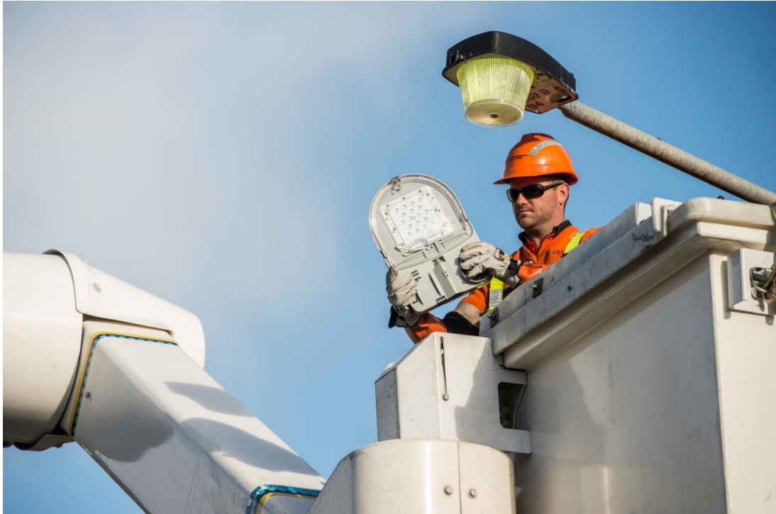
Replacement of Shoalhaven residential street lights with energy efficient LED lights in 2019/20.
