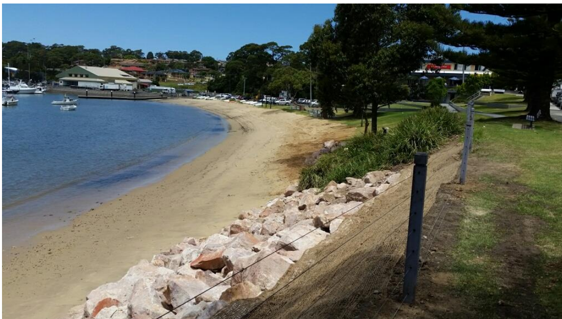
Figure 6-7 – Completed remediation works at Ulladulla Harbour
