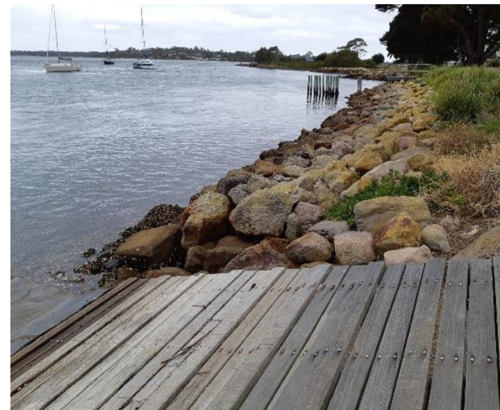
e) Example of foreshore protection works incorporating estuarine vegetation and timber kayak launching ramp, Greenwell Point
