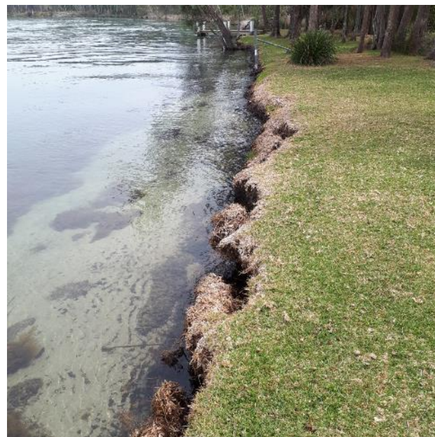
d) Bank erosion at Sussex Inlet
