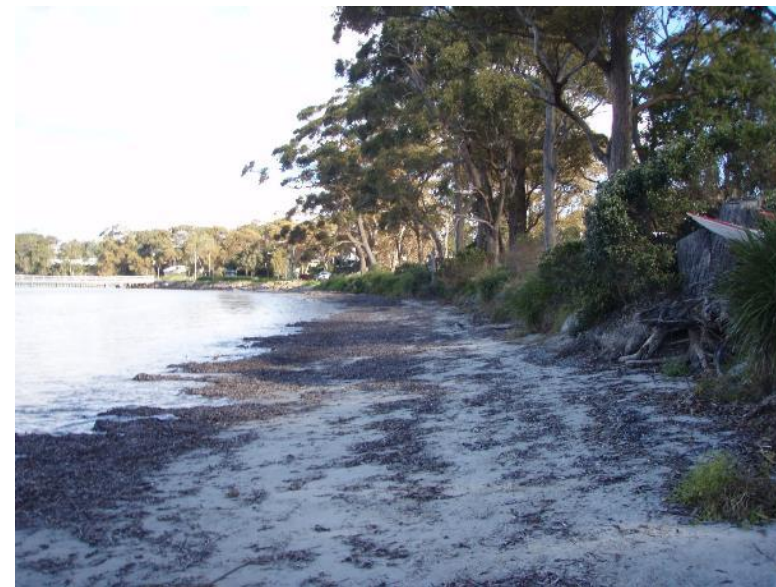
b) Foreshore erosion at Callala Bay.
