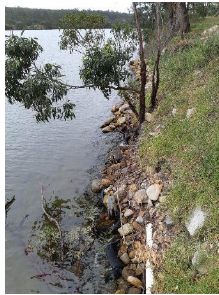
b) Ad-hoc foreshore protection works, Shoalhaven River.
