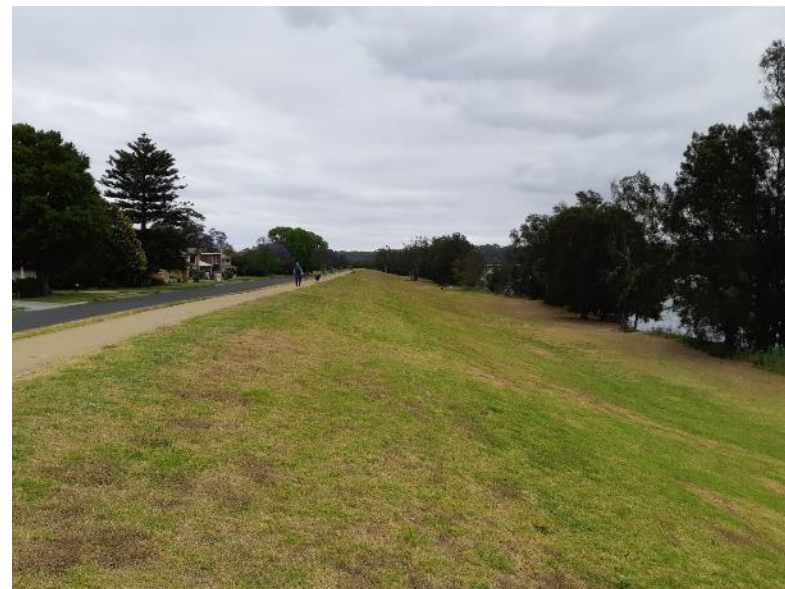
d) Flood levee to protect against flooding, Shoalhaven River Nowra
