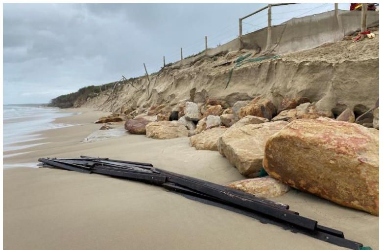
Erosion of sand dunes following storm, Shoalhaven Heads, January 2023.
