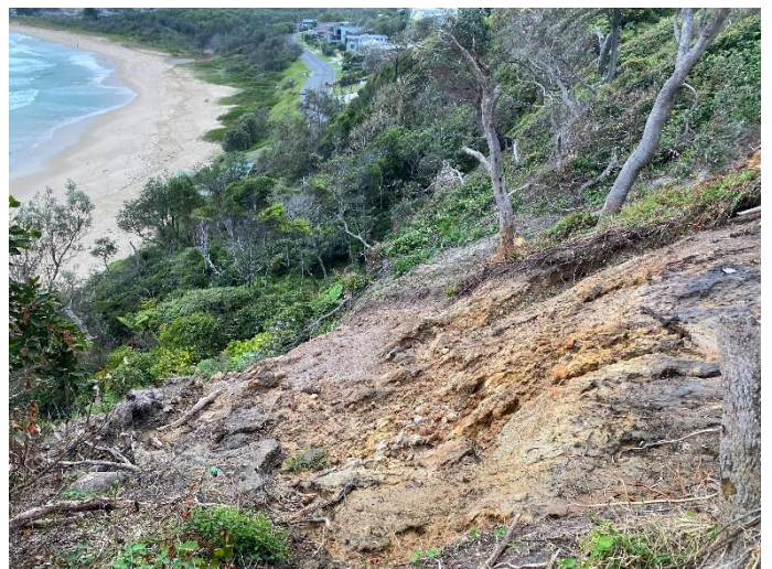
Coastal cliff instability at Bannister Head, March 2022. Mollymook Beach.
