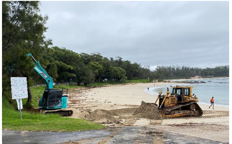
Machinery moving sand during NABE activities at Bendalong Beach, March 2022.
