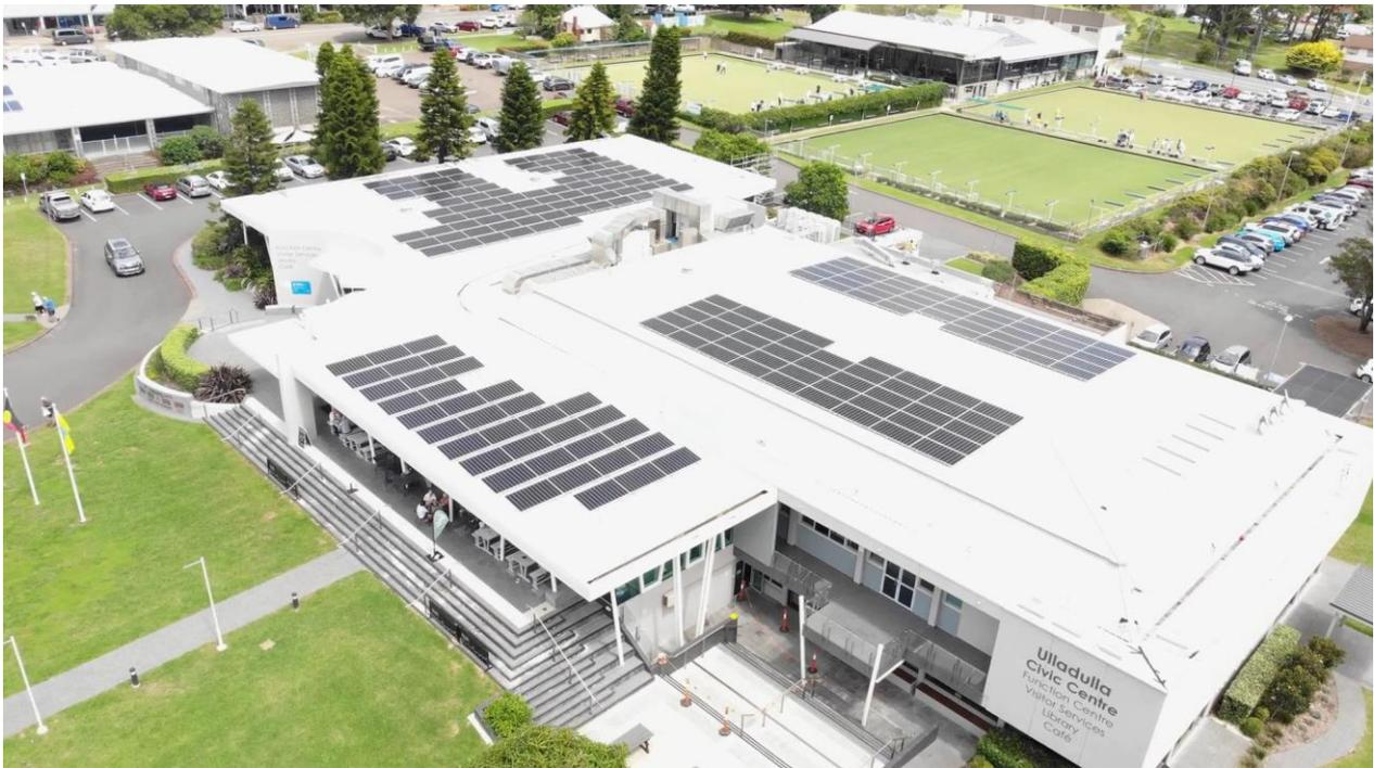
*A 100-kW solar PV system installed on the Ulladulla Civic Centre roof in 2023*
