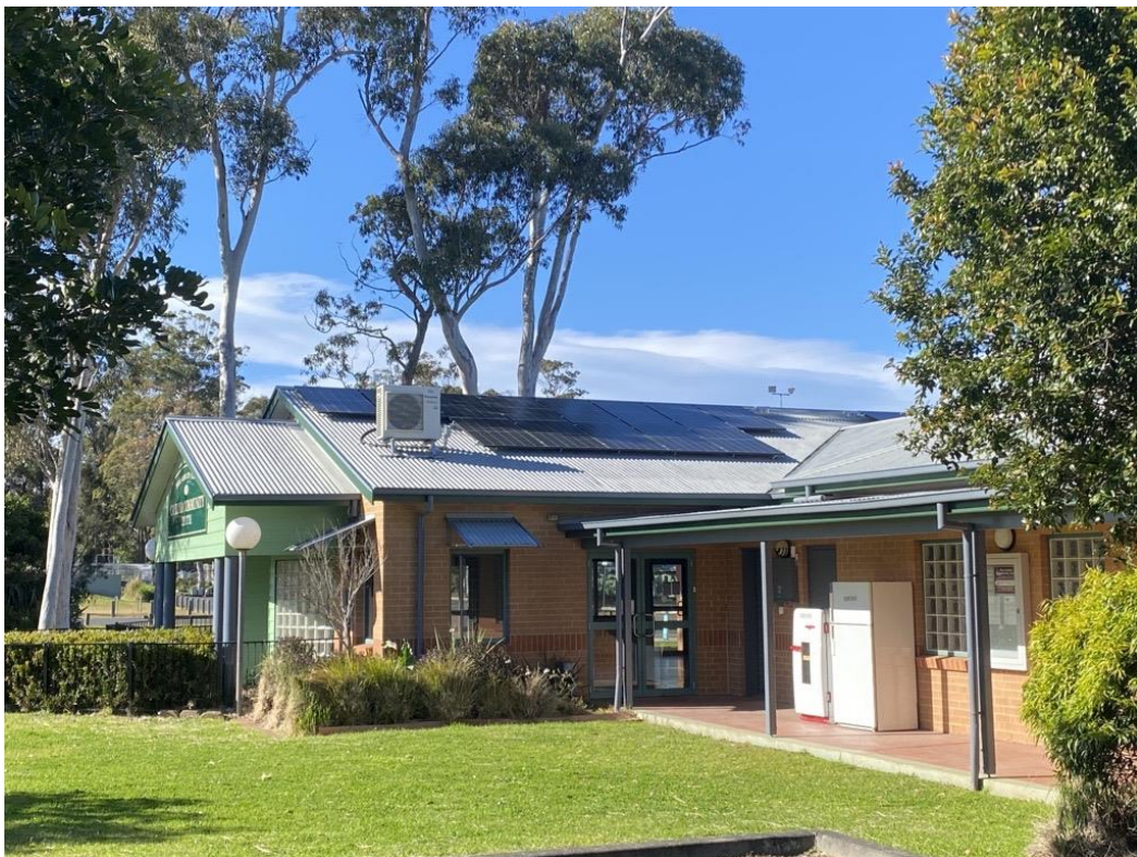
Solar PV installation at Calla Bay Community Hall under the Recovery into Resilience project
