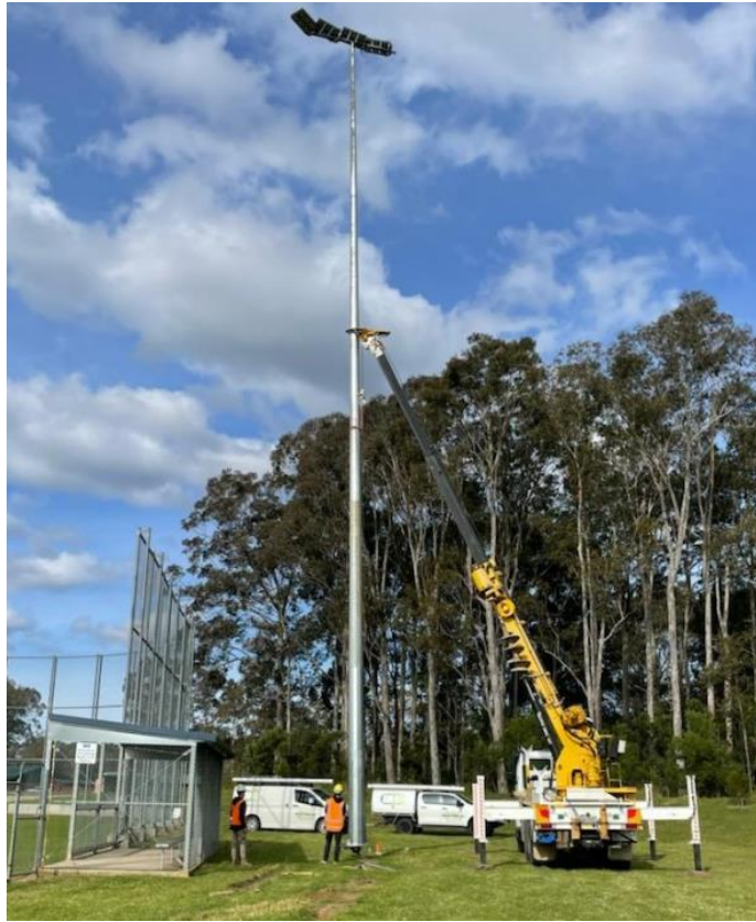
Energy savings LED flood lights being installed at Ison Park
