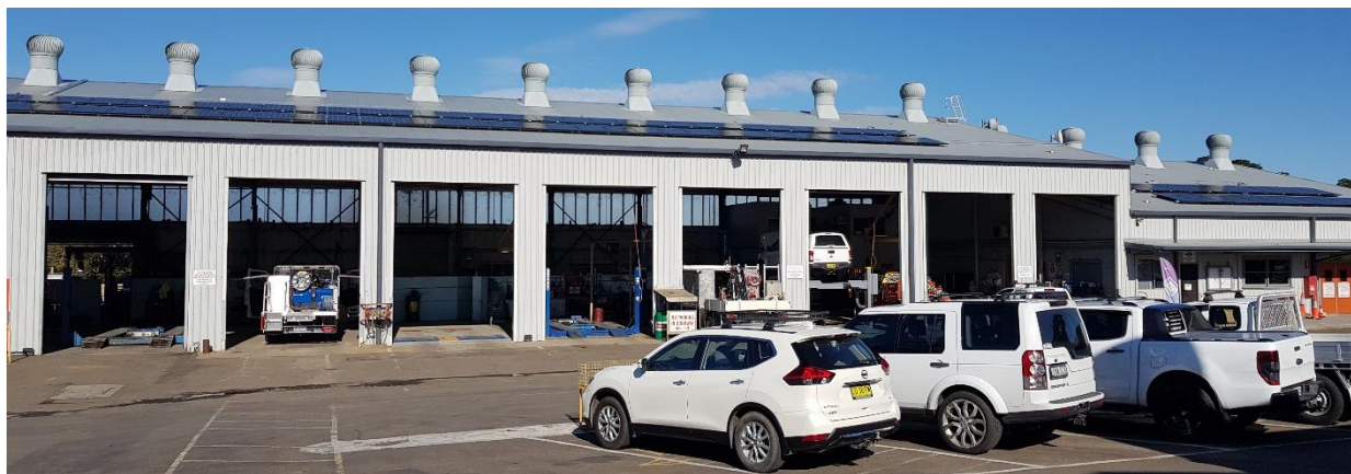
A 31 kW solar PV system installed on the rooftop of the Automotive Workshop at Shoalhaven Council's Bomaderry Works Depot in mid-2020
