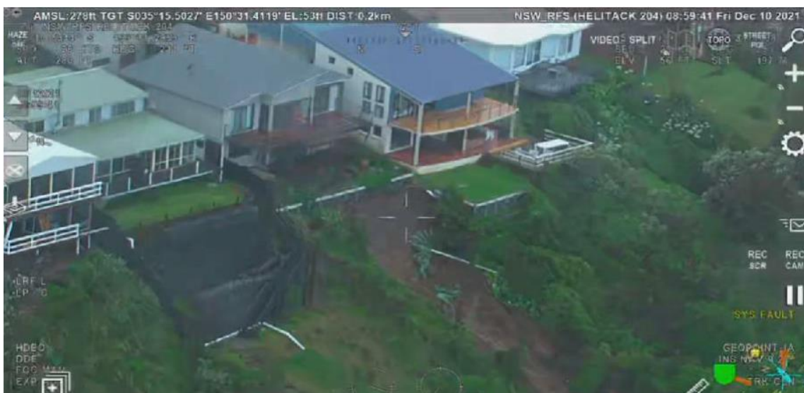
Figure 2-11 Coastal cliff and slope instability event at Inyadda Point following heavy rainfall in December 2021. (Douglas Partners, 2023)
