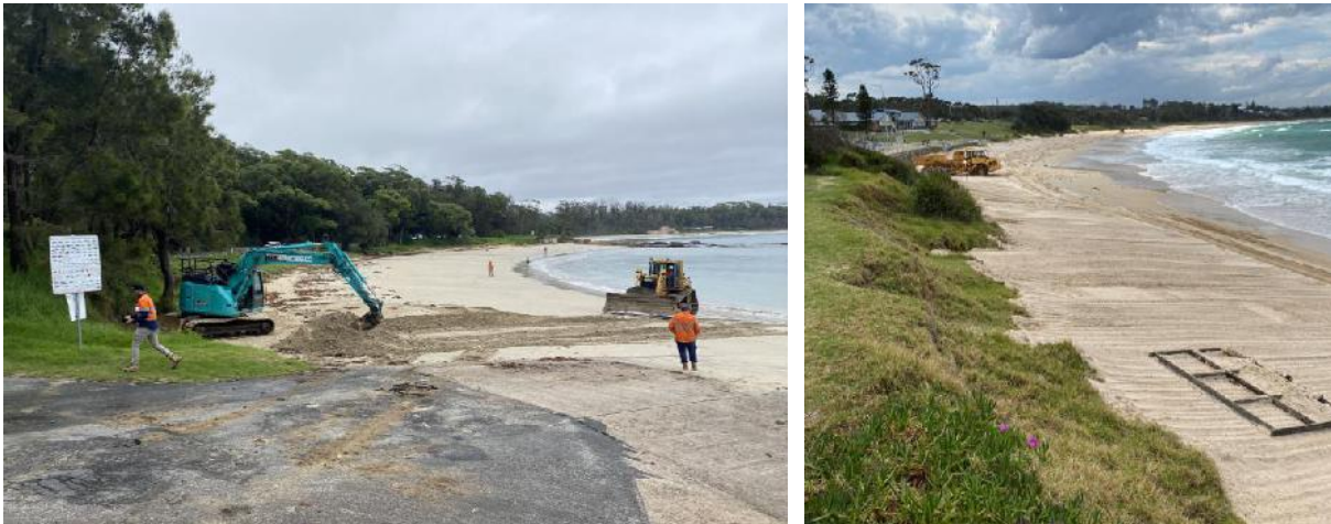
Figure C-1 Emergency beach scraping works undertaken by Council after storm events. Left: Bendalong Boat Harbour, April 2022. Right: Mollymook Beach, June 2020. Image source: SCC
