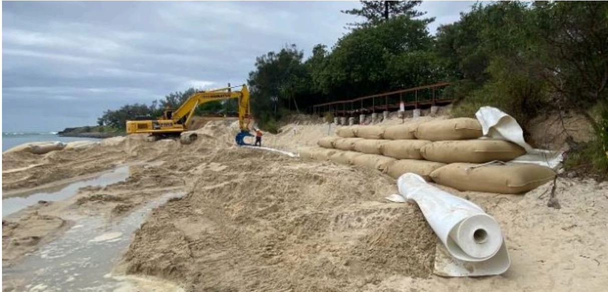
Figure C-6 Example of Interim 'Soft Works' in the Form of Temporary Geotextile Sand Containers. Photo Sourced from Mulcahey et al (2023)
