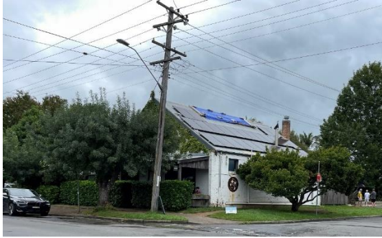
Figure 14. 23 Prince Alfred Street on the corner of Princess Street.
