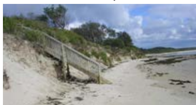
One of the staircases destroyed at Currarong.
