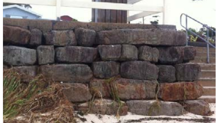
Voids in the sea wall have opened further (above) and a corner section collapsed (below) during the ECL.
