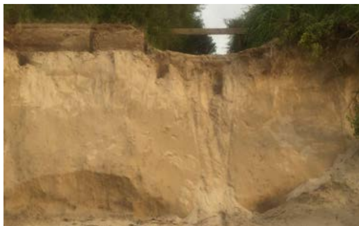
Imprints in the sand—all that was left of a viewing platform and staircase at the eastern end of Currarong Beach.
