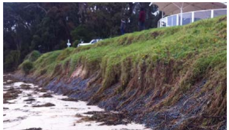
Each time the gabions are exposed, further damage is done.
