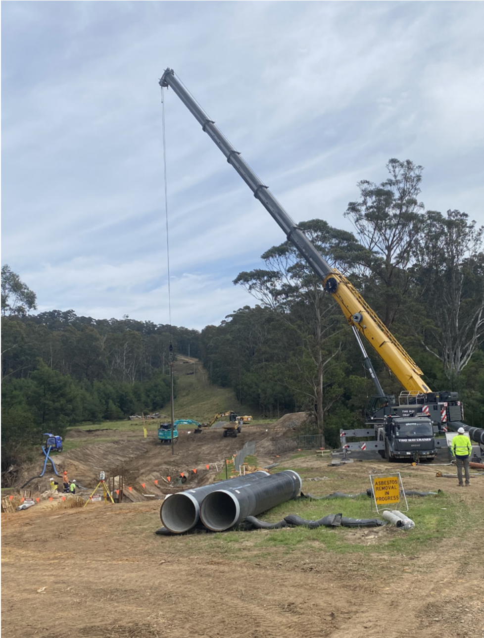
Water pipeline work on track
