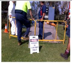
4.14.2.2 Confined Space work sites accessed on a regular basis will have the below Danger Confined Space sign installed at each entry point.
