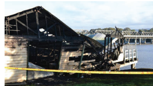
The damaged building following the 2017 fire (source: South Coast Register)
