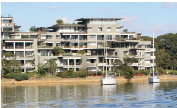
Development with a range of heights from 2 to 4 along the water and up to 7 storeys behind which creates interest and allows view sharing
