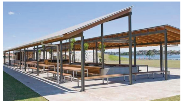
Shaded public seating under a lightweight structure
