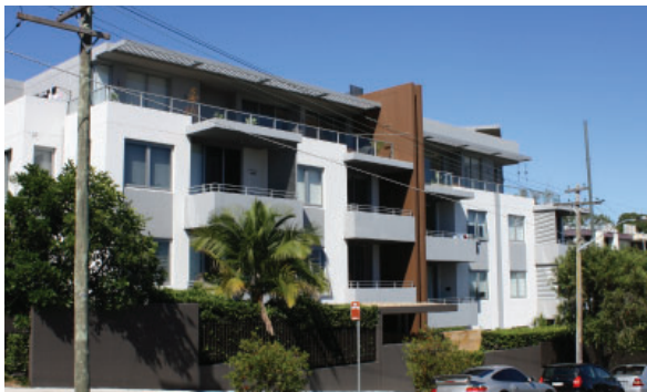
Development stepping down to follow the slope of 3-4 storeys high with an upper floor setback.
