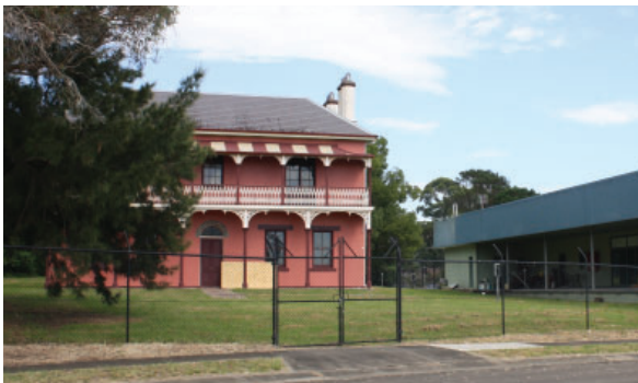
The state heritage listed Graham Lodge is a key component of this sub-precinct and a key consideration for any future development.
