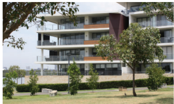
4 storey development along the waterfront at Rhodes with large elevated terraces providing surveillance of the open space.
