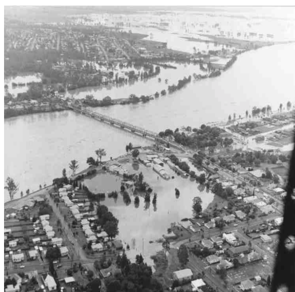
Photo 1: Nowra Bridge and Civic Centre Site - March 1978 Flood
