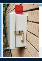
Turn off the sound of the alarm by pressing the mute button underneath the alarm panel. The alarm light will continue to be activated.
