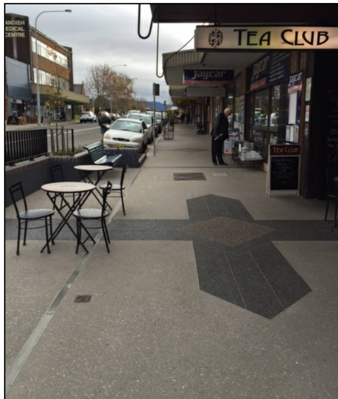
Specially Designed Aggregate & Resin Footpath Pattern
