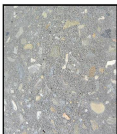
Honed Concrete Surface Finish
