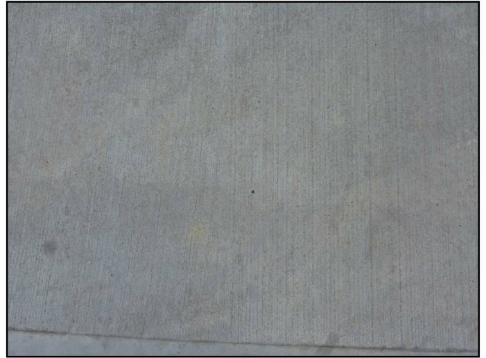
'Colormix' "Bluestone" with R10 non-slip broom finish
