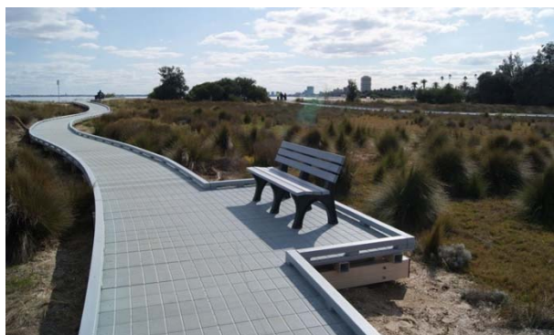
Raised recycled composite boardwalk
