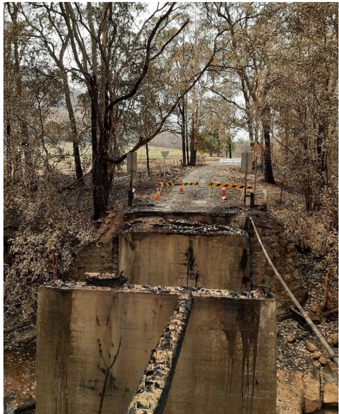
Figure 4: Burnt out School Creek Bridge, Budgong (Source: Shoalhaven City Council)
