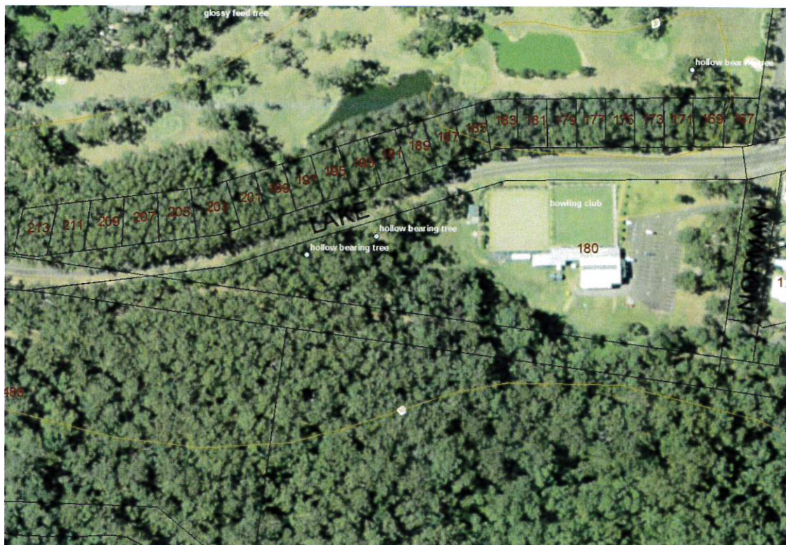
Figure 7: Hollow-bearing trees located in the western portion of the alignment to be retained and protected during construction
