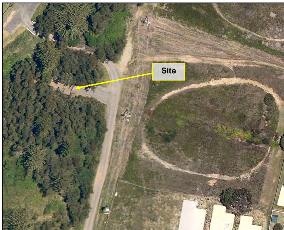
Figure 7: Aerial photo of Culburra SPS 10.
