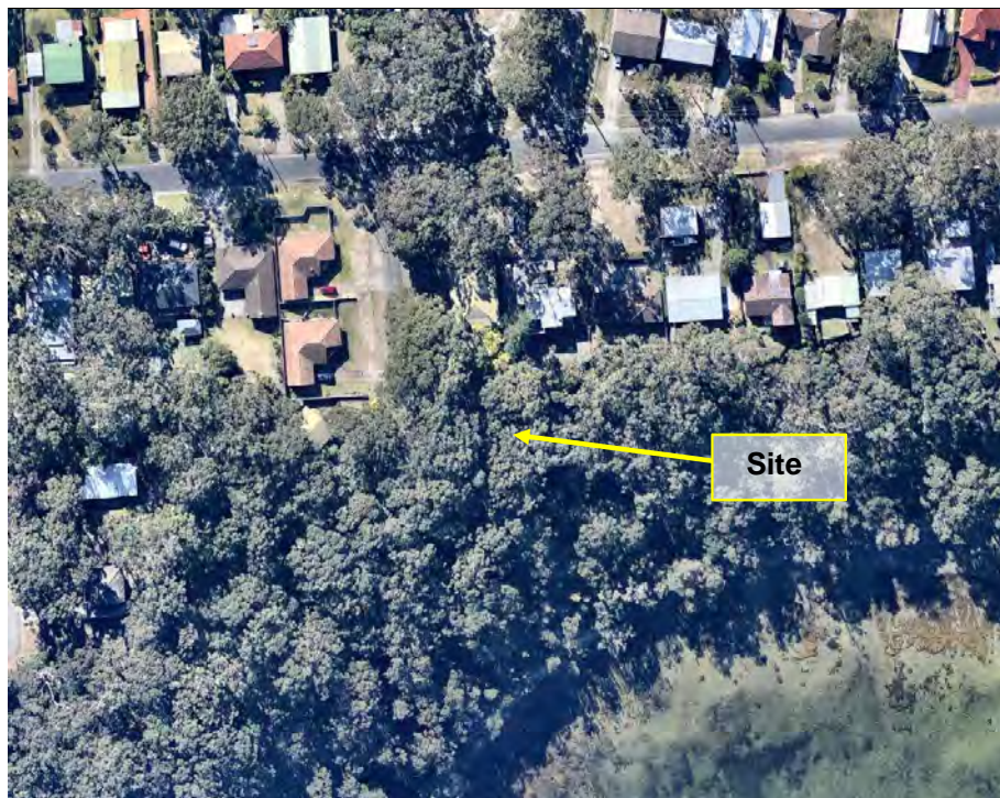
Figure 13: Aerial photo of St Georges Basin SPS 13.
