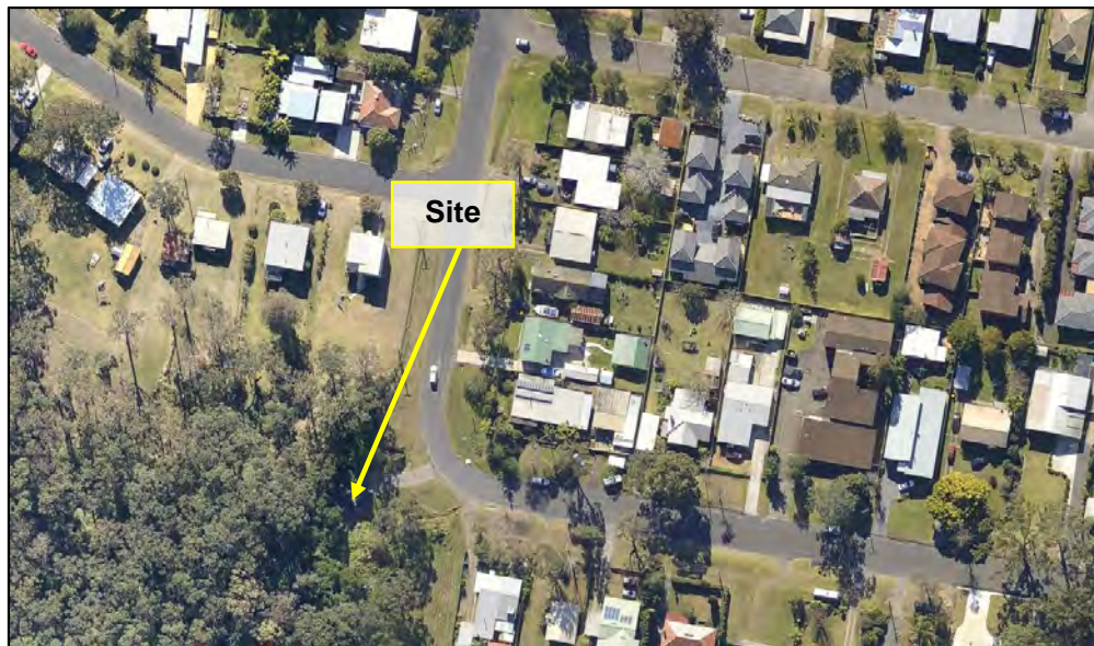
Figure 9: Aerial photo of Huskisson Vincentia SPS 3.
