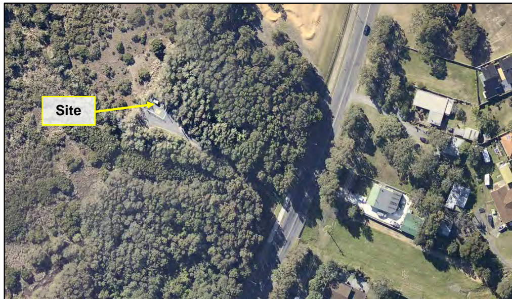
Figure 5: Aerial photo of Culburra SPS 6.
