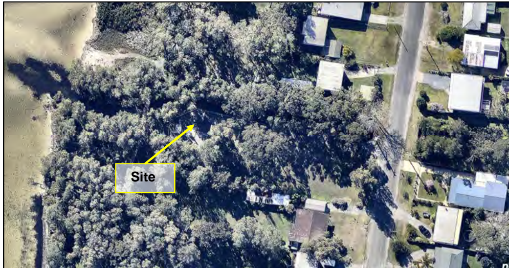
Figure 12: Aerial photo of St Georges Basin SPS 12.
