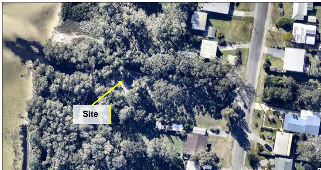
Figure 12: Aerial photo of St Georges Basin SPS 12.
