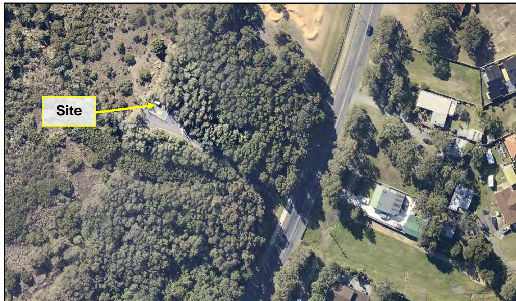
Figure 5: Aerial photo of Culburra SPS 6.
