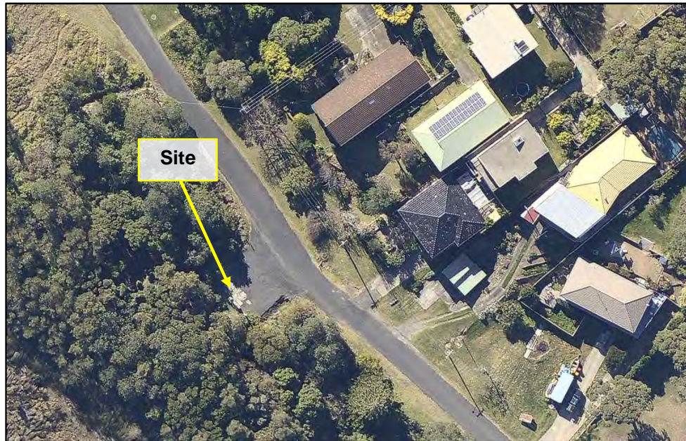
Figure 6: Aerial photo of Culburra SPS 9.
