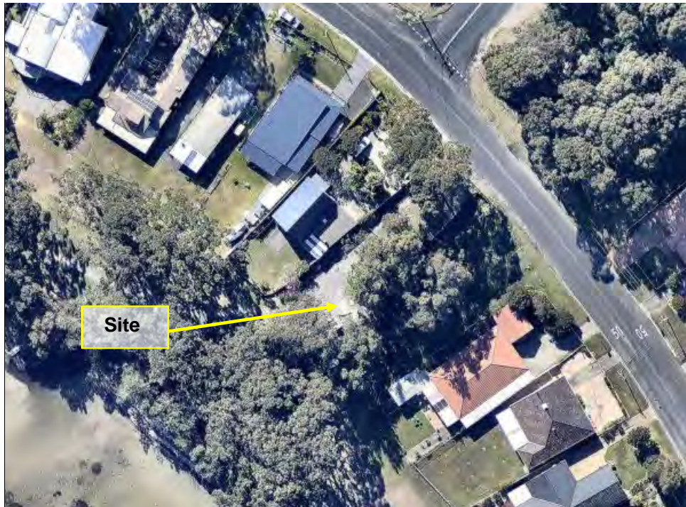
Figure 11: Aerial photo of St Georges Basin SPS 10.
