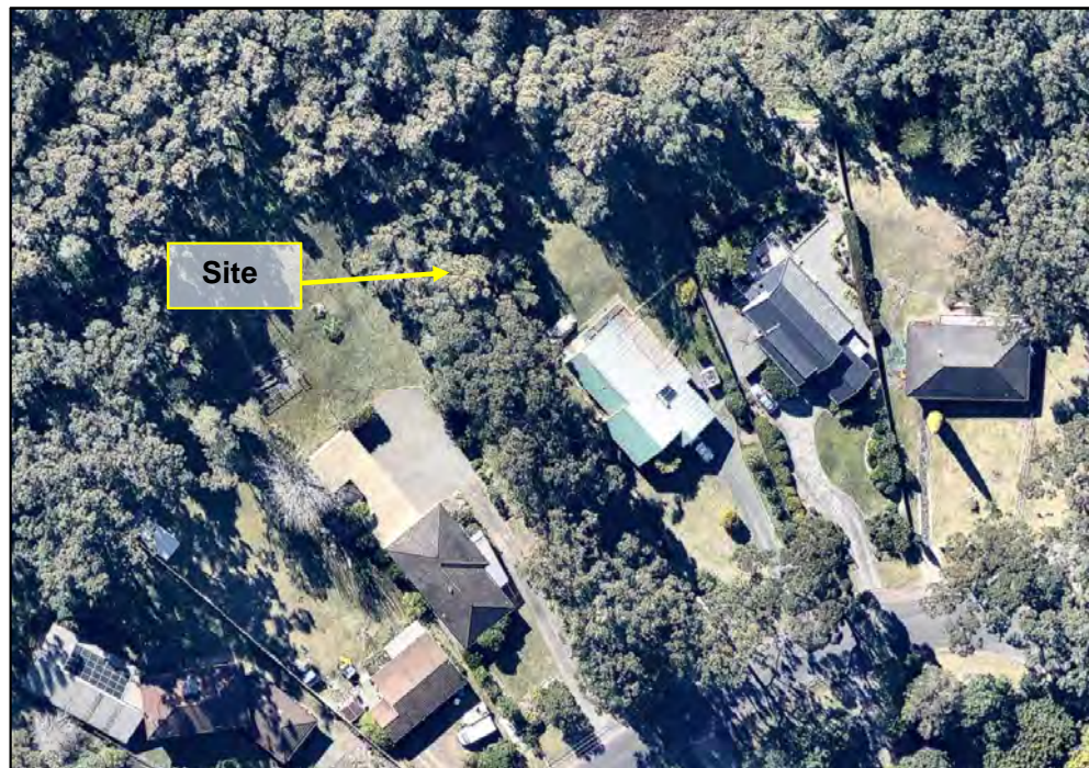
Figure 16: Aerial photo of Sussex Inlet SPS 1.
