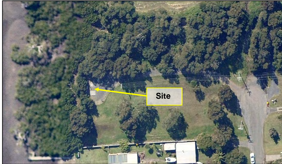
Figure 4: Aerial photo of Culburra SPS 5.
