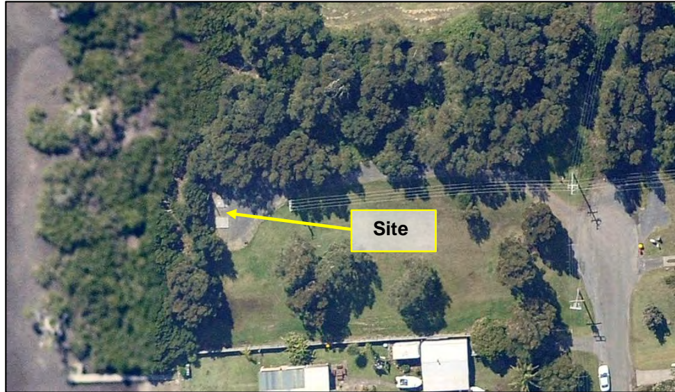
Figure 4: Aerial photo of Culburra SPS 5.
