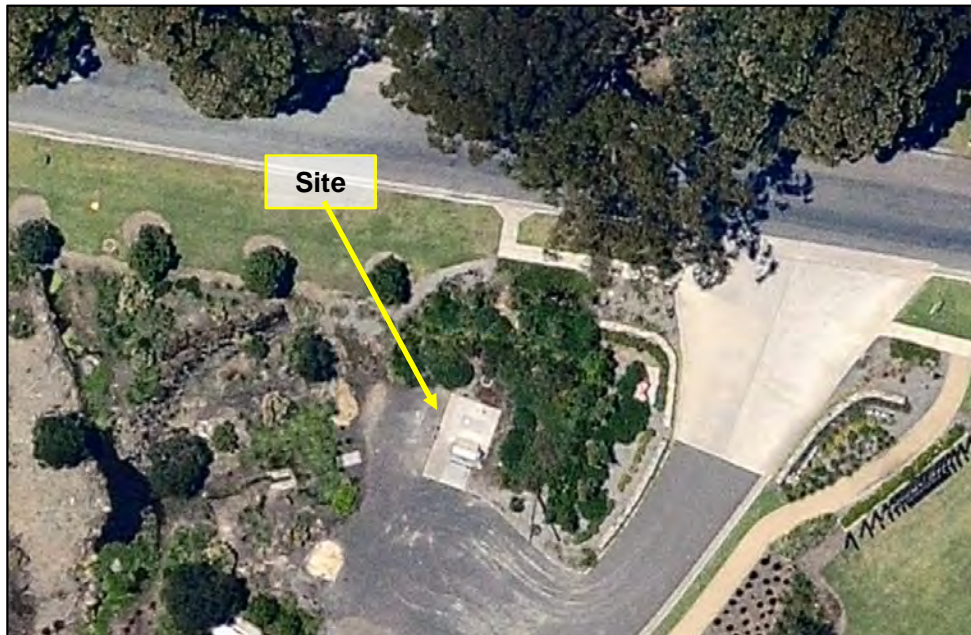
Figure 2: Aerial photo of Berry SPS 5.
