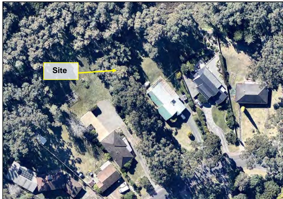
Figure 16: Aerial photo of Sussex Inlet SPS 1.
