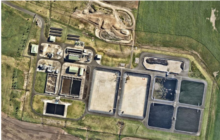
Figure 4-2 – Photograph of Nowra Sewage Treatment Plant
