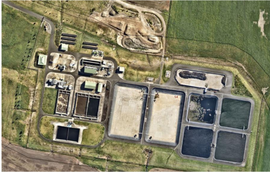
Figure 4-2 – Photograph of Nowra Sewage Treatment Plant
