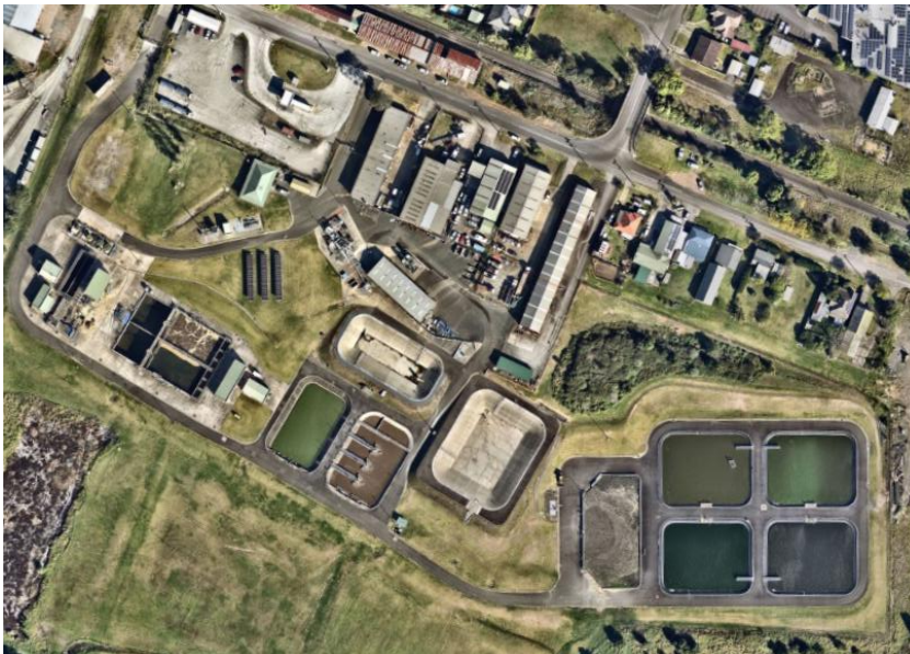
Figure 4-1 – Photograph of Bomaderry Sewage Treatment Plant
