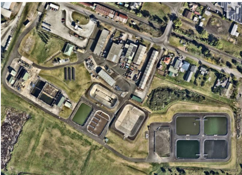
Figure 4-1 – Photograph of Bomaderry Sewage Treatment Plant
