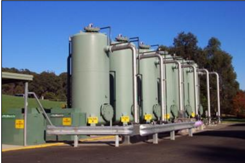
Figure 2-2 – Photograph of Filters Callala WwTP
