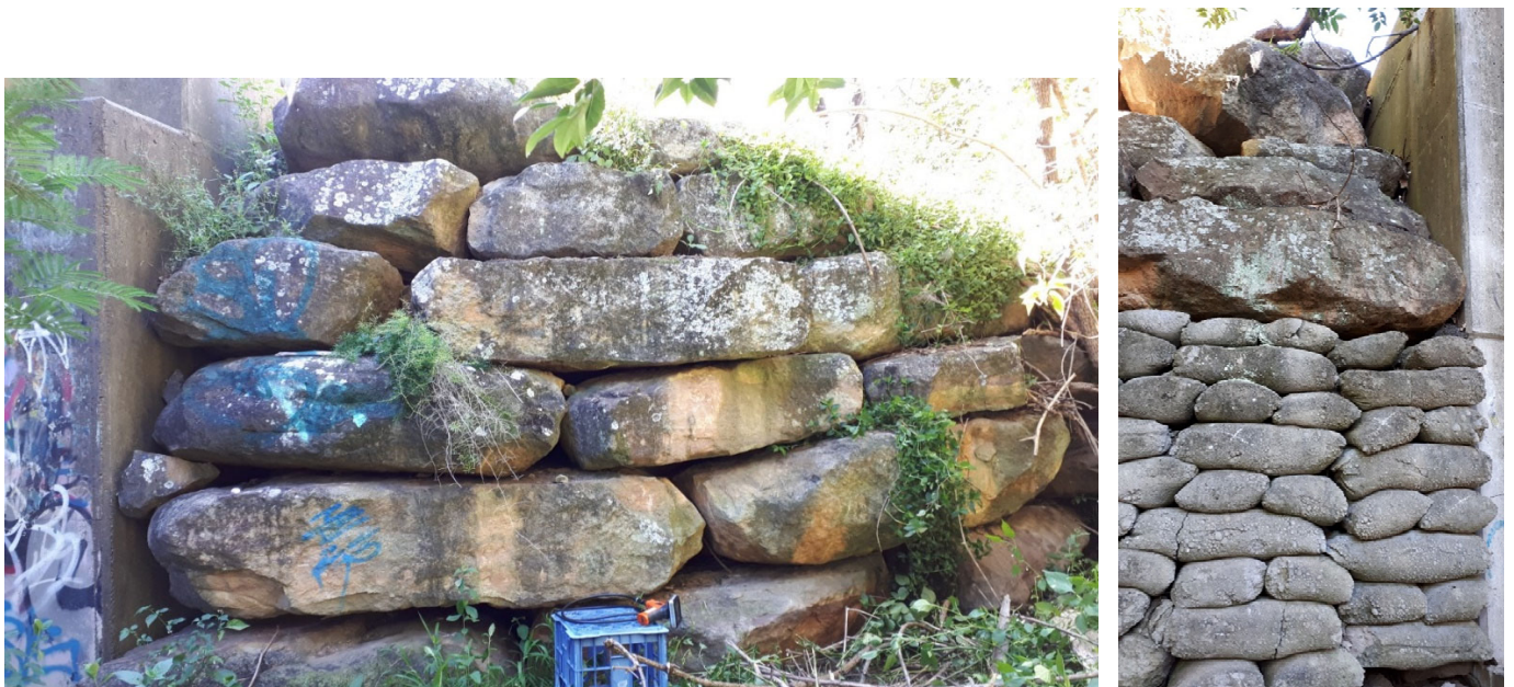
Photo 8. Rock scour protection on the southern side of Good Dog Creek bridge
