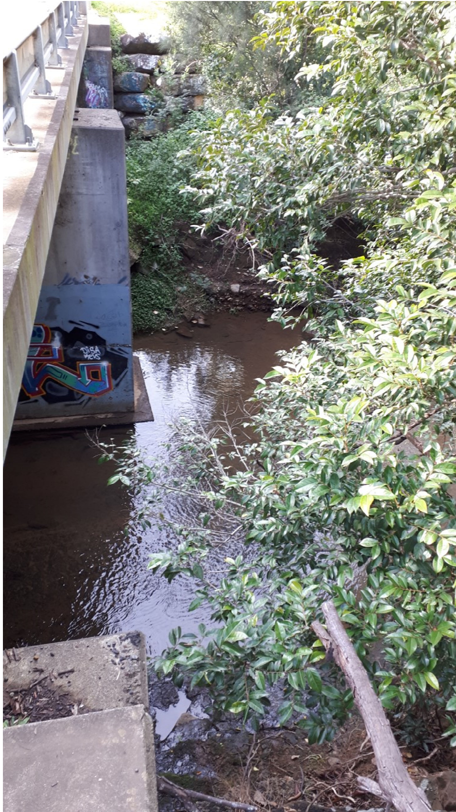
Photo 2. Southern side of Good Dog Creek bridge facing east, showing rock scour protection
